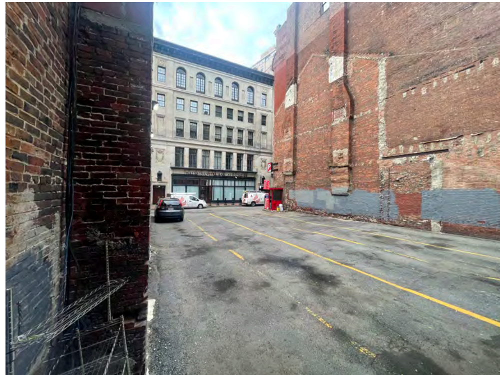
Back Left Corner of 17-23 West St looking towards the street
