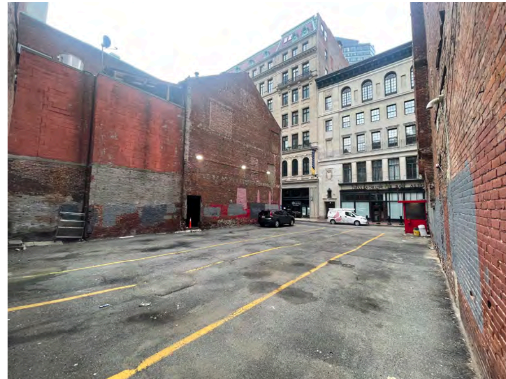
Back Right Corner of 17-23 West St looking towards the street
