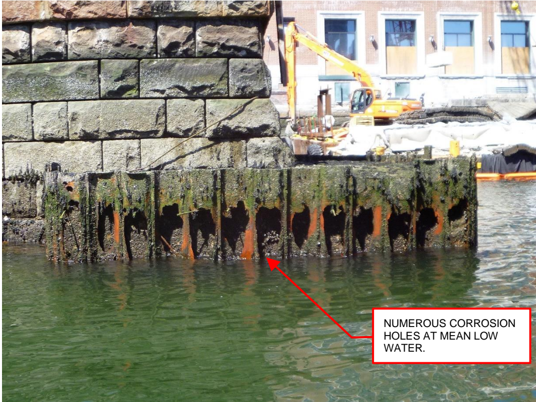
Photo 15 – Corrosion holes in steel sheet pile for concrete encasements.
