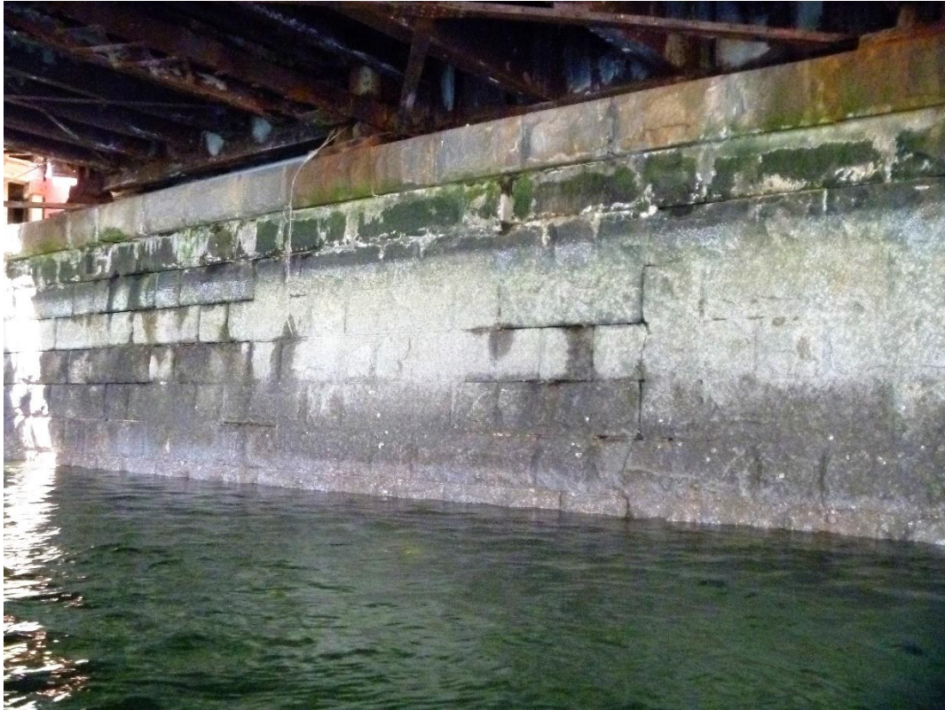
Photo 1 – Overall view of the Boston Abutment, looking northwest.
