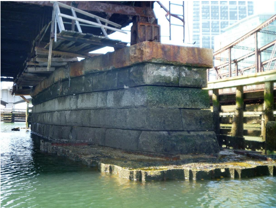
Photo 4 – Overall view of Pier 2, looking west.
