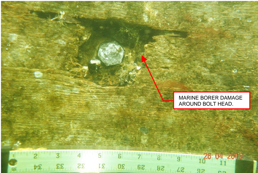
Photo 24 – Typical timber wale connection below water.
