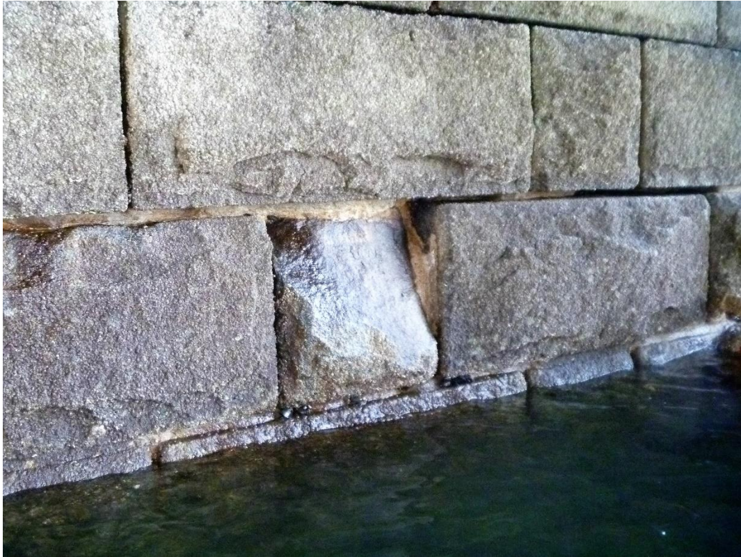
Photo 13 – Cleaved corner of granite block in Pier lower course.
