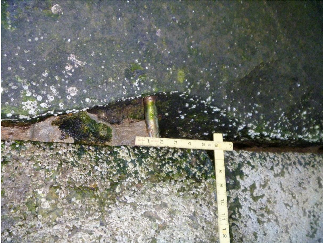
Photo 11 – Exposed stainless steel tie rod in granite block of Pier 2's East face.
