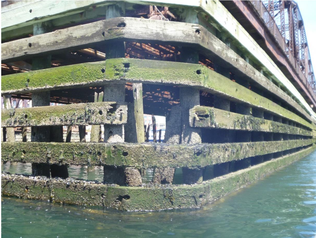
Photo 25 – Missing timber wale section at south corner of West Fender System.
