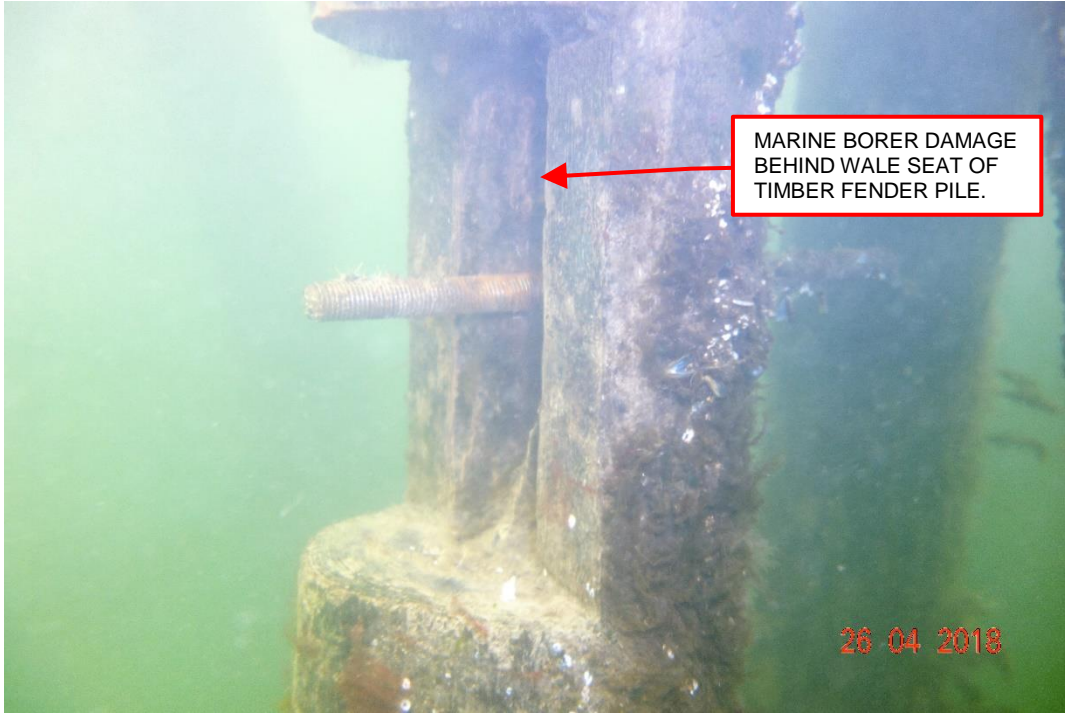
Photo 27 – Separated section of timber wale for the Fender System.
