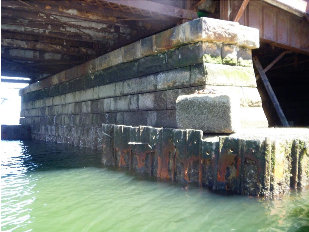
Photo 5 – Overall view of Pier 3, looking east.
