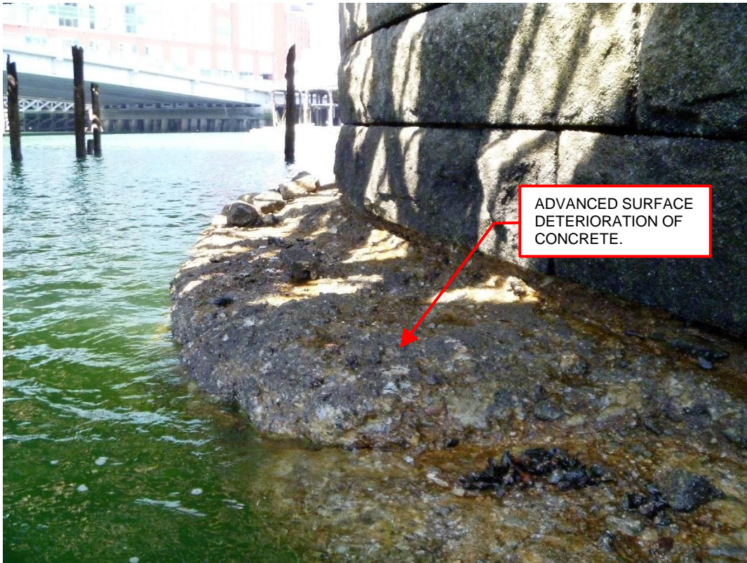
Photo 16 – Top of concrete footing near southwest quadrant of the Draw Pier.
