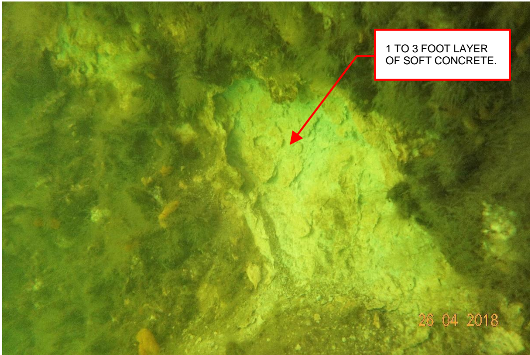
Photo 19 – Concrete footing for Draw Pier below water.
