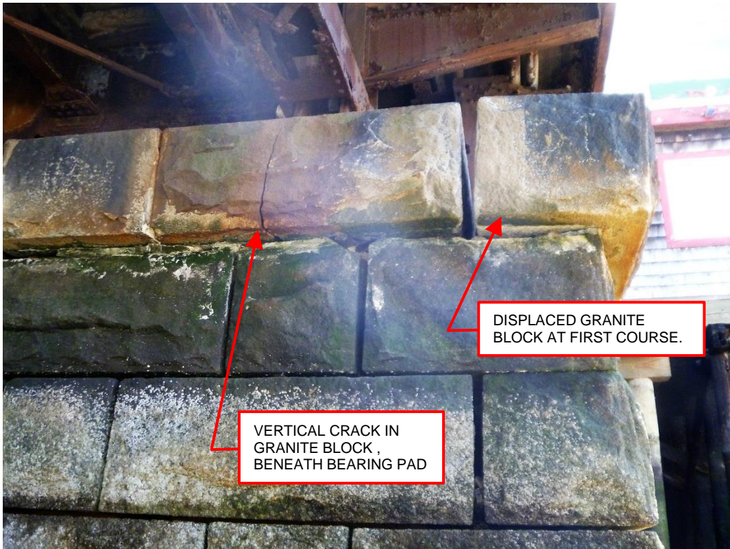
Photo 12 – Vertical crack in granite block, and displaced granite block.
