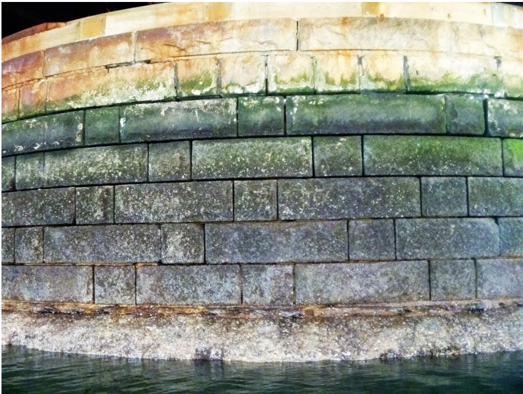
Photo 6 – View of the northeast quadrant of the Draw Pier, looking southwest.
