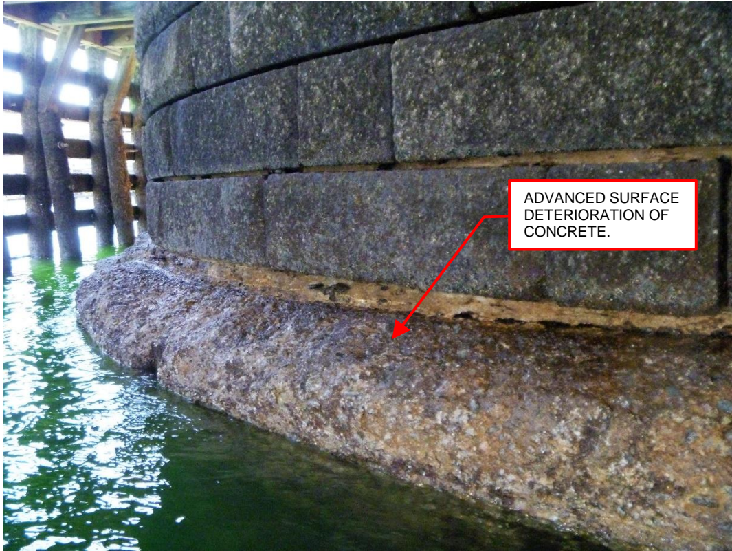
Photo 17 – Top of concrete footing near northeast quadrant of the Draw Pier.
