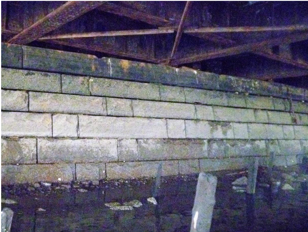
Photo 2 – Overall view of the South Boston Abutment, looking south.
