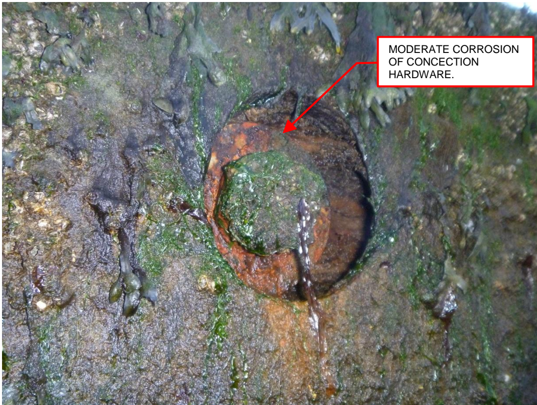
Photo 26 – Typical lower timber wale connection.
