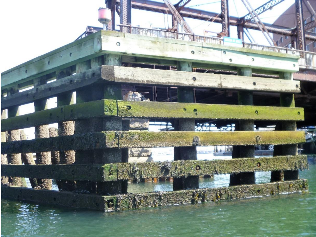
Photo 7 – View of the southwest end of the East Fender System, looking east.
