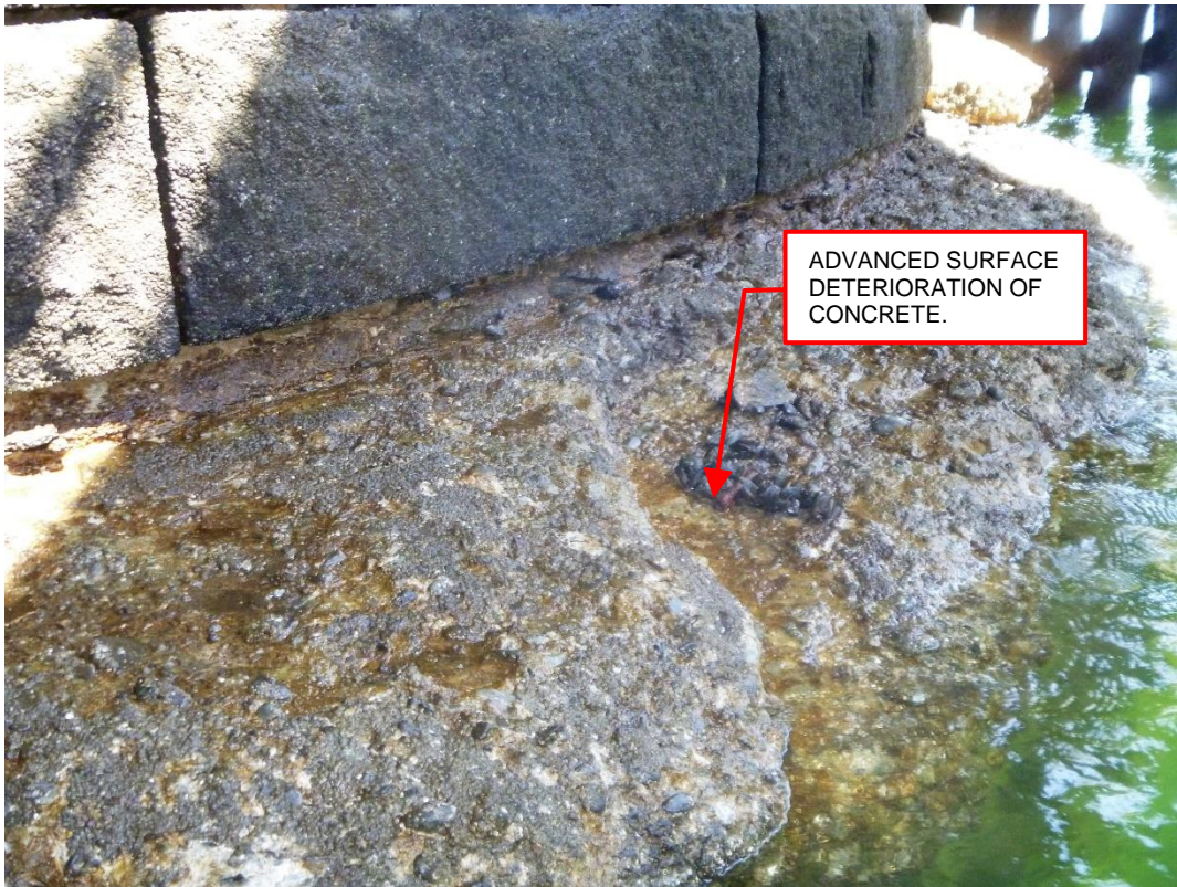
Photo 18 – Typical top of concrete footing for Draw Pier.
