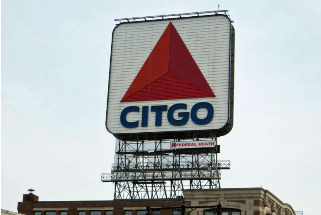
FIGURE 2.3.5 Close-up of the west face of the Citgo sign and supporting steel truss. Photo by Dayl Cohen
