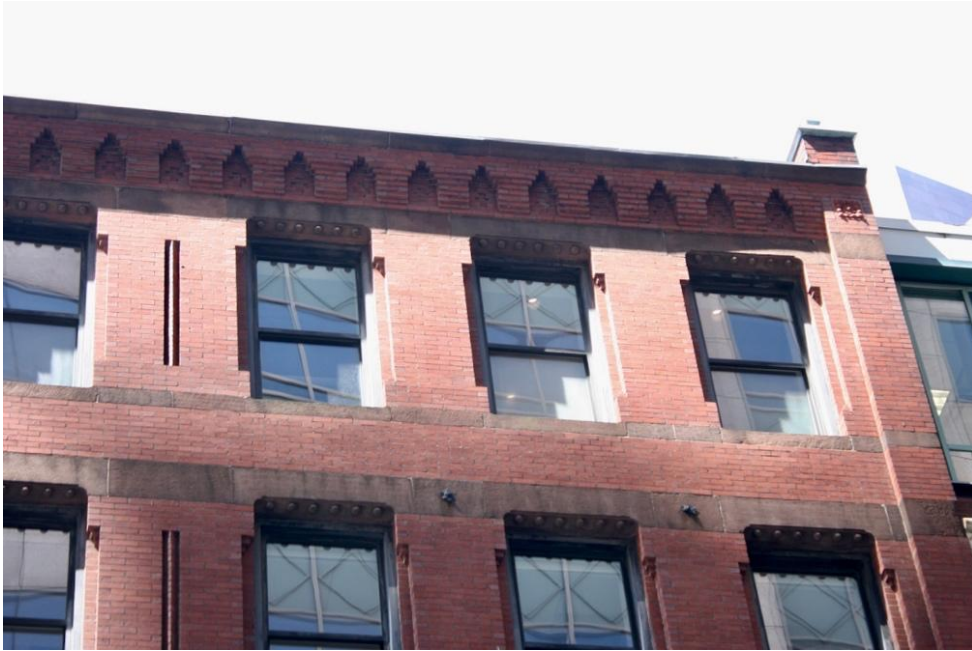
Figure 14. Upper levels and roof edge, 115-119 Pearl St. façade. Photograph by Wendy Frontiero, June 2023.
