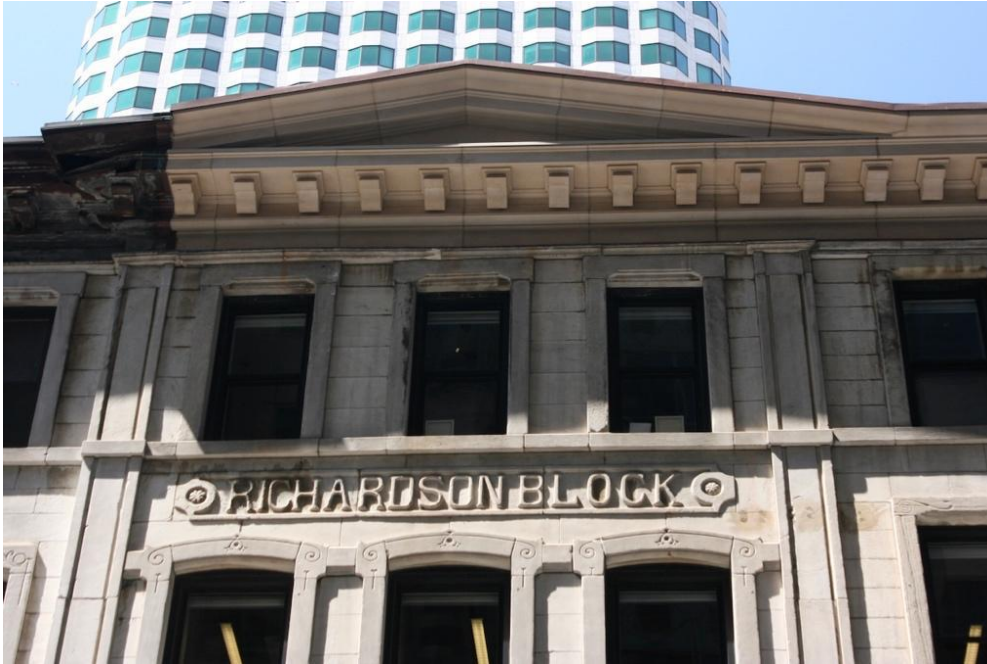
Figure 12. 129-131 Pearl St. façade, upper levels and roof edge. Photograph by Wendy Frontiero, June 2023.
