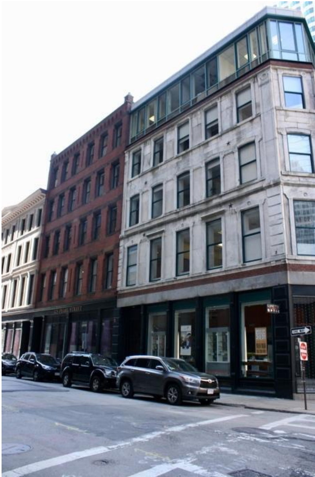
Figure 7. 115-119 Pearl St. and 119 High St. façades. Photograph by Wendy Frontiero, June 2023.
