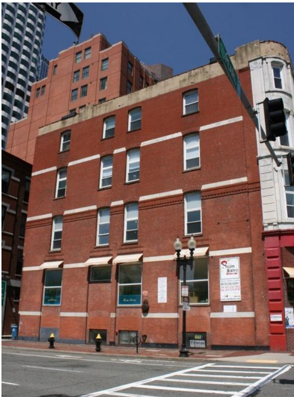
Figure 15. 149-151 Pearl St., Purchase Street elevation. Photograph by Wendy Frontiero, June 2023.
