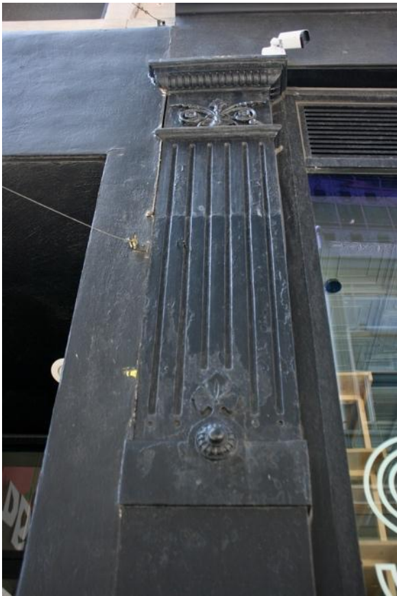
Figure 11. 129-131 Pearl St. storefront detail. Photograph by Wendy Frontiero, June 2023.
