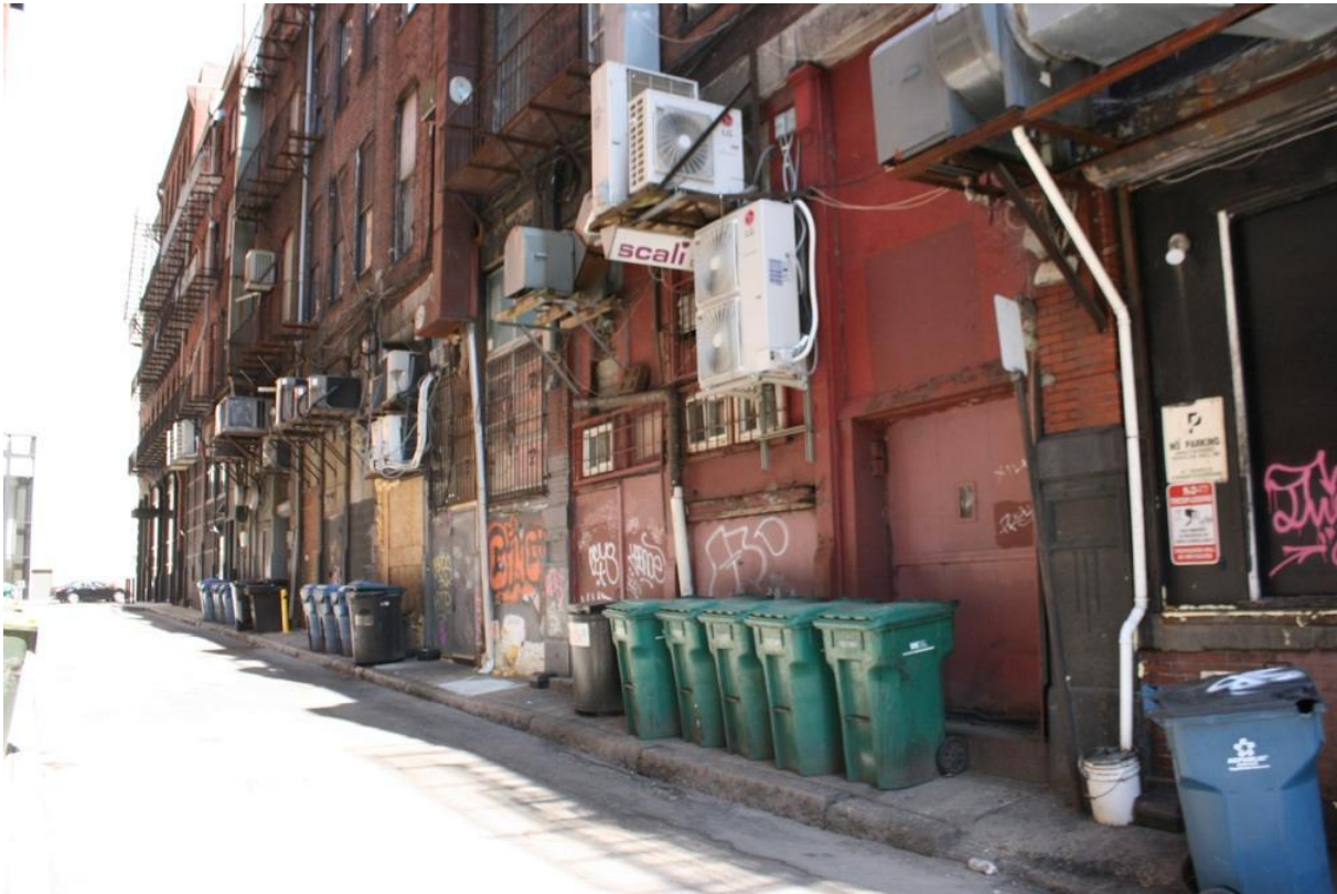
Figure 19. Gridley Street elevations, looking toward High Street. Photograph by Wendy Frontiero, June 2023.
