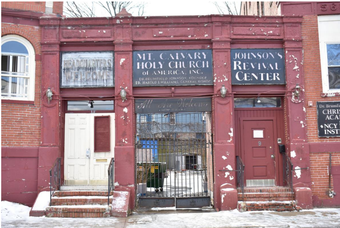
Photo 2. Entrance, Roxbury Hebrew School and Congregation Sharei Tfila/Mt. Calvary Holy Church, 9-13 and 15 Otisfield Street, looking southwest.
