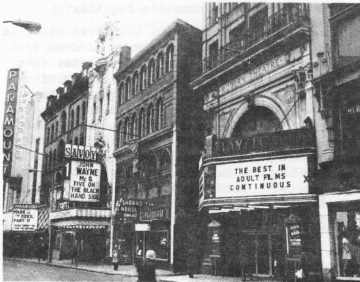
Washington Street before the Savoy was converted to the Opera House in 1978. Photo courtesy of the Boston Landmarks Commission.
