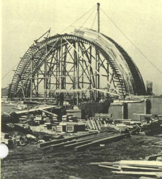
1939 - Hatch Shell Construction Credit: Laning Humphrey
