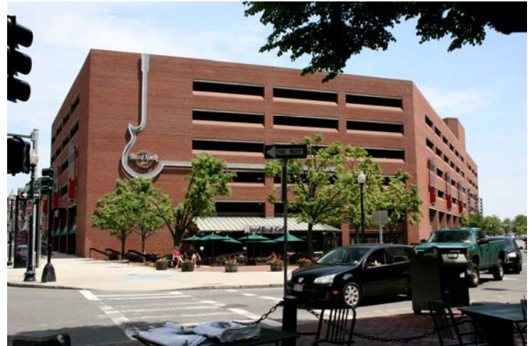
North, west, and south facades (North and Clinton streets)
