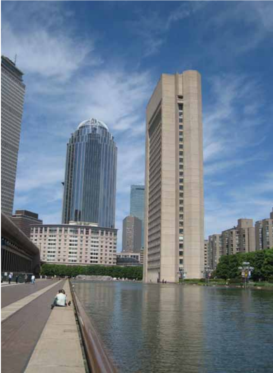
The length of the Reflecting Pool punctuated by the height of the Administration Building Photo courtesy of Boston Preservation Alliance
