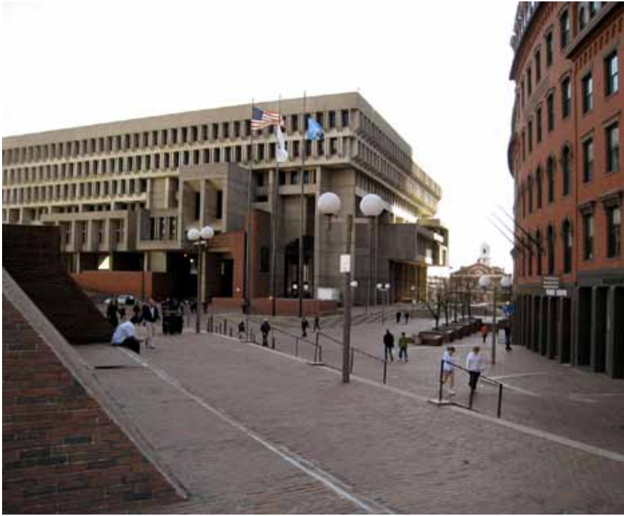
Boston's City Hall Plaza's Grade Changes Photo courtesy of Boston Preservation Alliance
