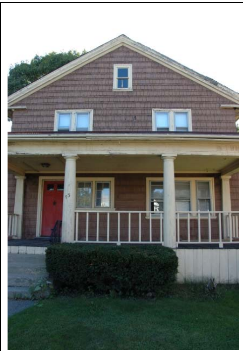
Rectory, entrance facade
