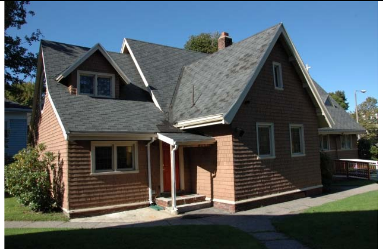
Chapel, with 1916 addition at rear
