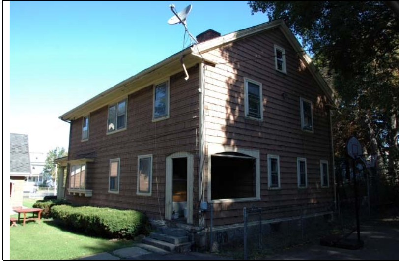
Rectory, SE elevation
