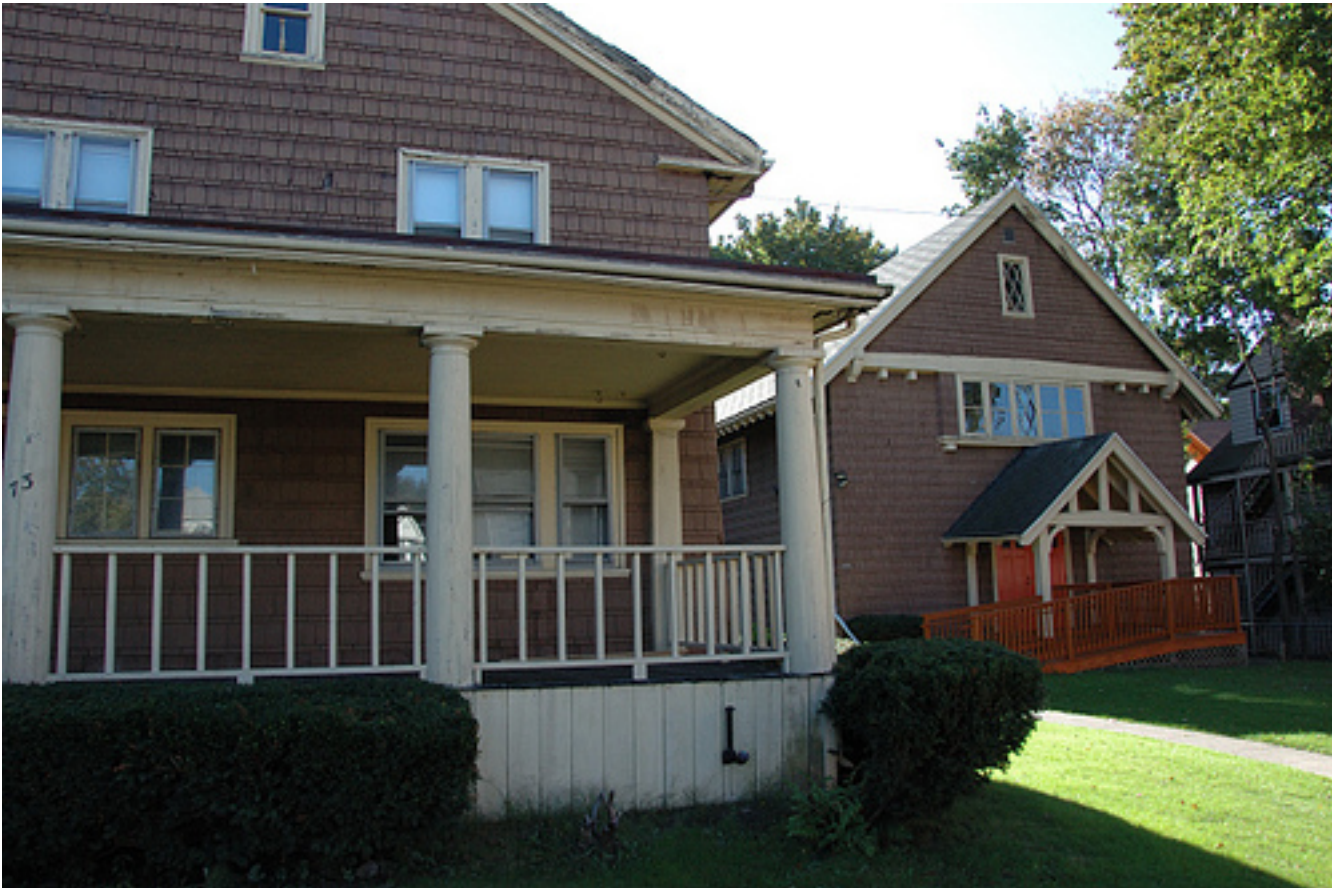
Figure 1: The rectory (left) (BOS.13995) and the parish hall (right) (BOS.13996). Both buildings were constructed to the rear of the chapel (1904) at 73 Columbia Road in 1909.
