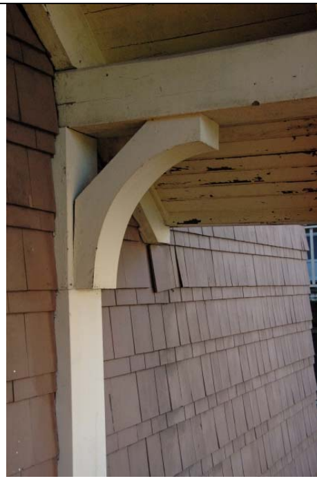
Parish hall, detail of front entrance
