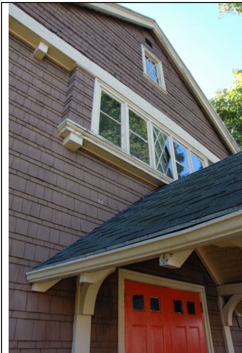
Entrance to Parish Hall (1909)
