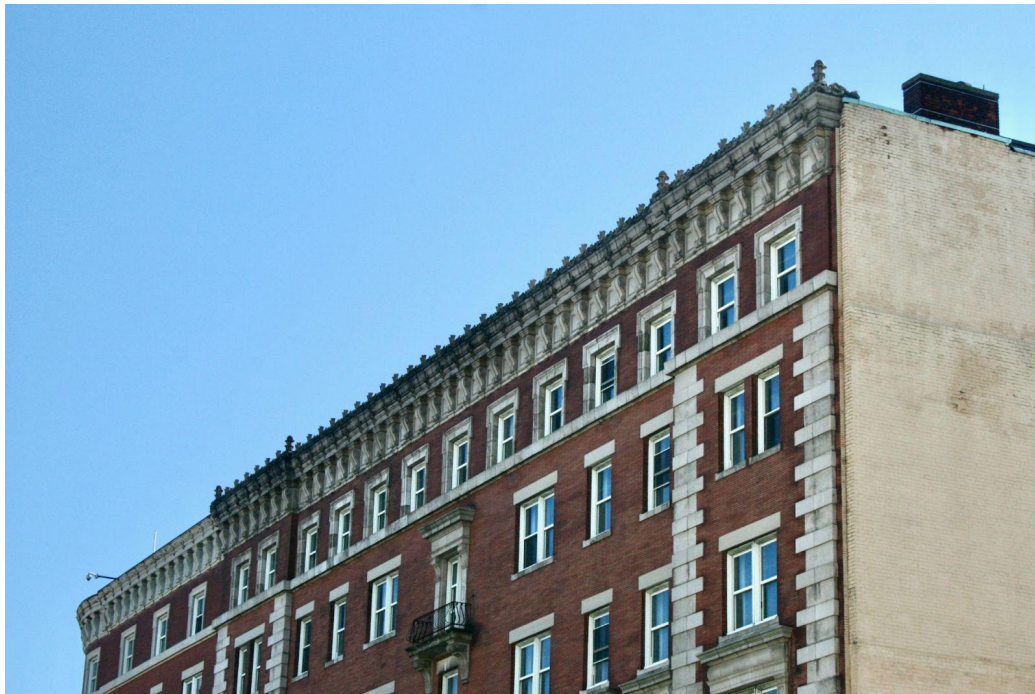
Figure 5. Beacon Street elevation, entablature detail. October 2022.
