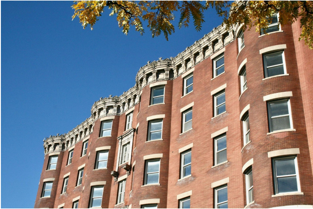
Figure 10. Brookline Avenue elevation, detail of bow windows. October 2022.
