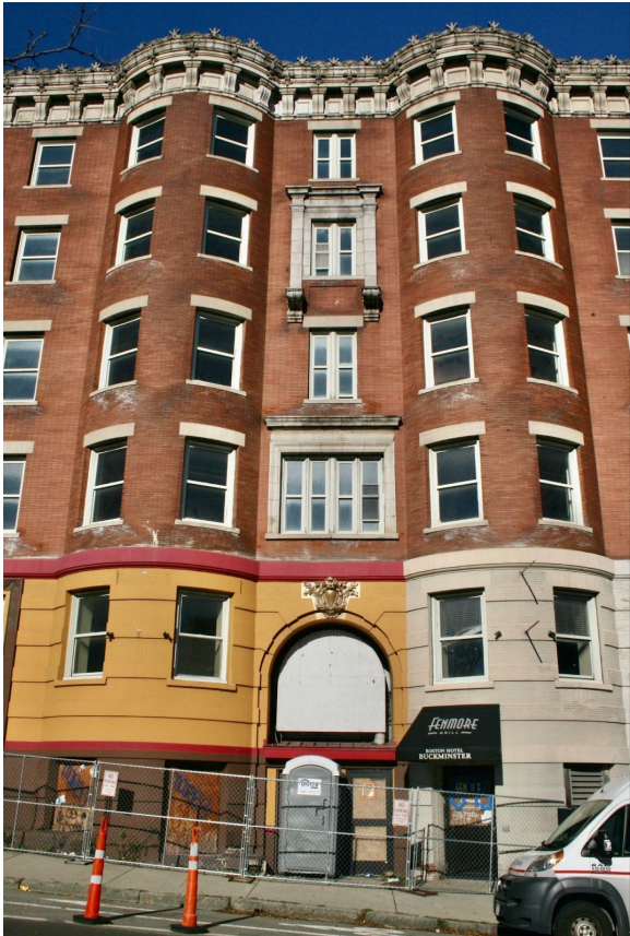
Figure 11. Brookline Avenue elevation, detail of main entrance bay. October 2022.
