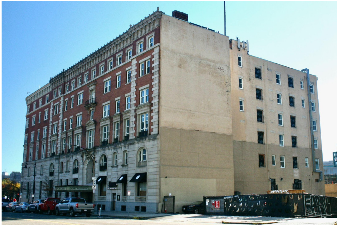
Figure 13. Beacon Street (left) and southwest elevations, view east. October 2022.
