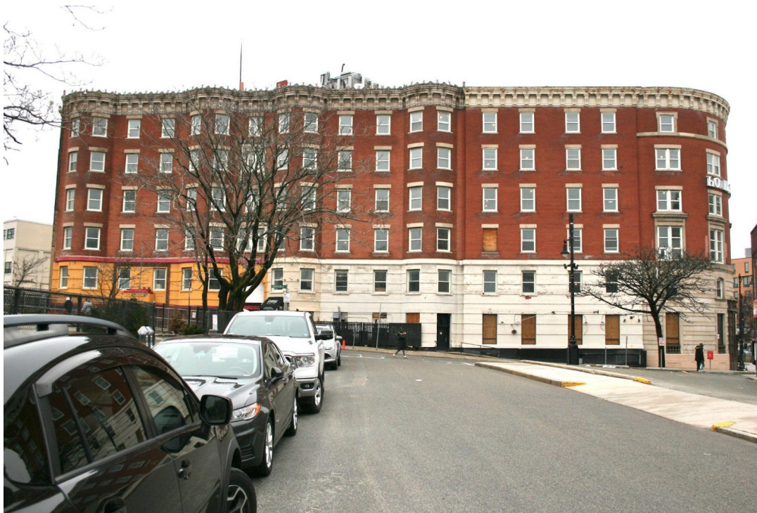
Figure 9. Brookline Avenue elevation, view northwest from Newbury Street. March 2023.
