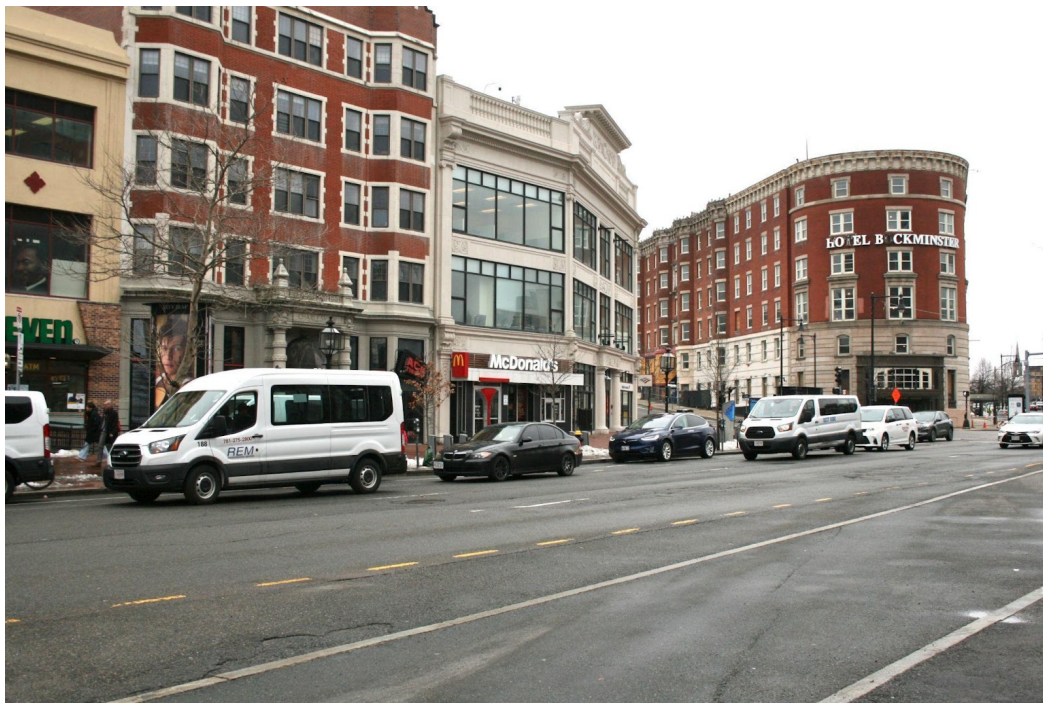
Figure 7. View southwest from Commonwealth Avenue. March 2023.
