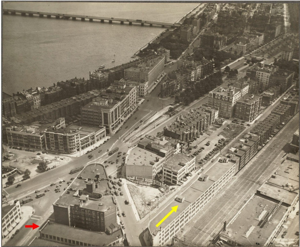
Figure 16. Aerial view (1929) northeast through the Kenmore Square area, showing the Hotel Buckminster in the left foreground. The building abutting the southwest elevation of the Buckminster (red arrow), demolished in 2003, is shown at its original one-story height. All buildings lining the south side of Newbury Street (yellow arrow) would be demolished ca. 1963 for construction of the Massachusetts Turnpike Extension.
