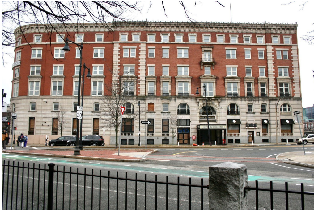
Figure 2. Beacon Street elevation, view southeast from Commonwealth Avenue. March 2023.
