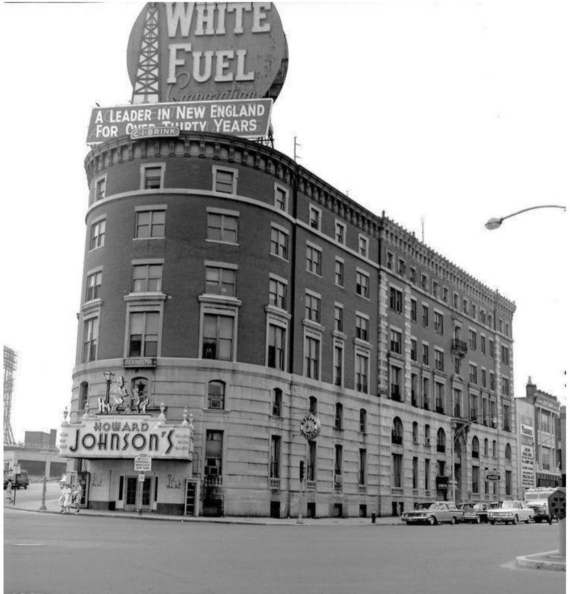
Figure 19. Undated (early 1960s) view south from Commonwealth Avenue, showing neon signs of Howard Johnson's restaurant and White Fuel Corporation on Kenmore Square elevation. Image from Boston Public Library.
