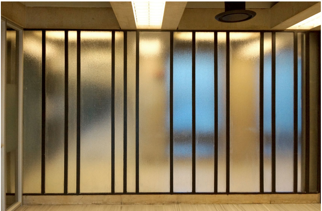
The storefront system at the eighth-floor municipal level (January 26, 2021).
