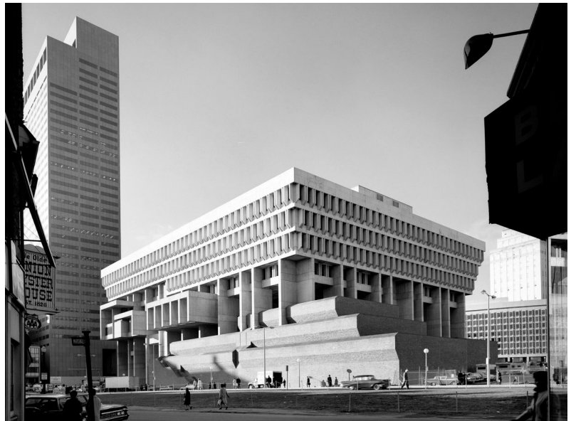
Bottom: View of the east and north elevations from the Union Oyster House.
