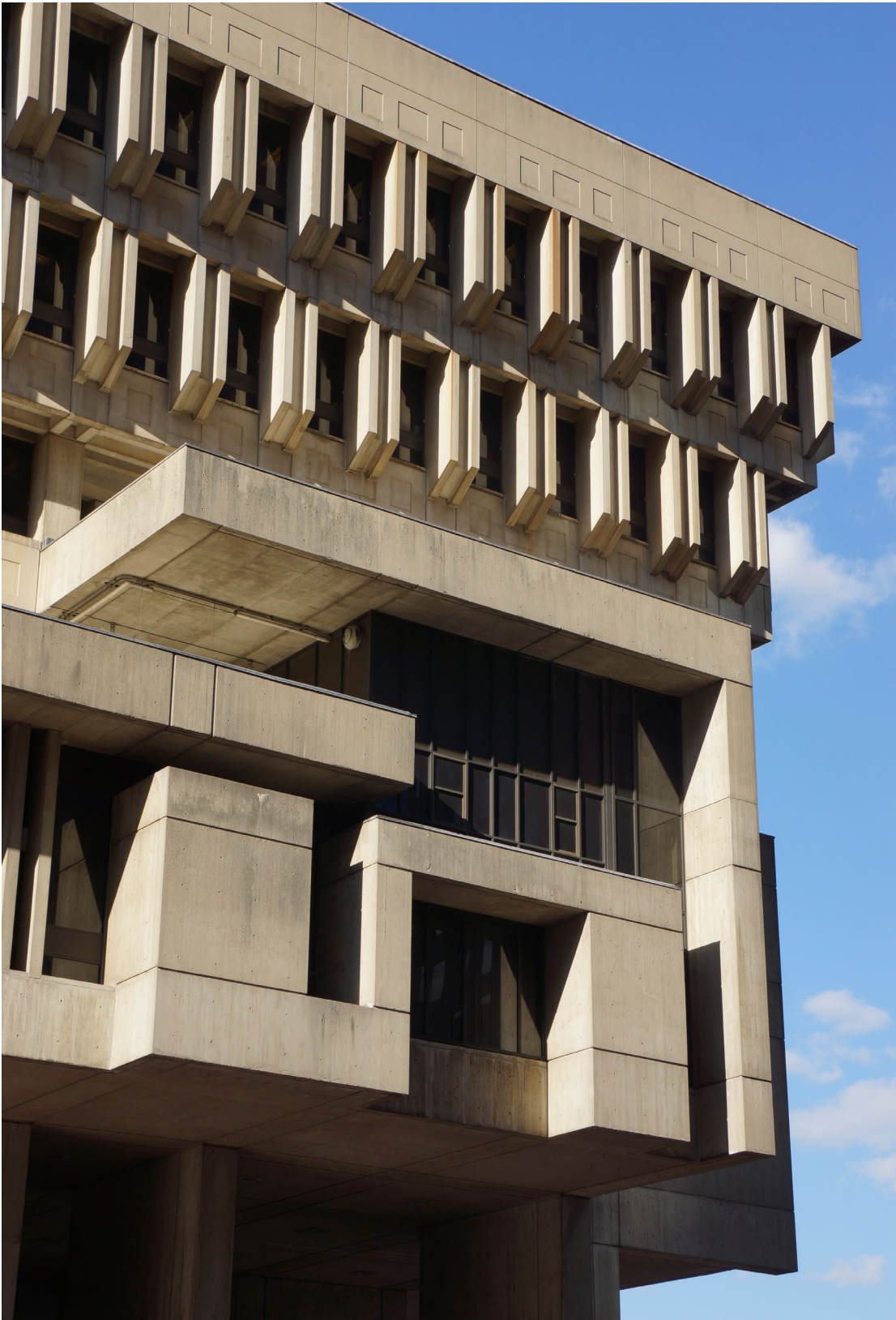
View of the southeast corner and mayor's office suite hoods.
