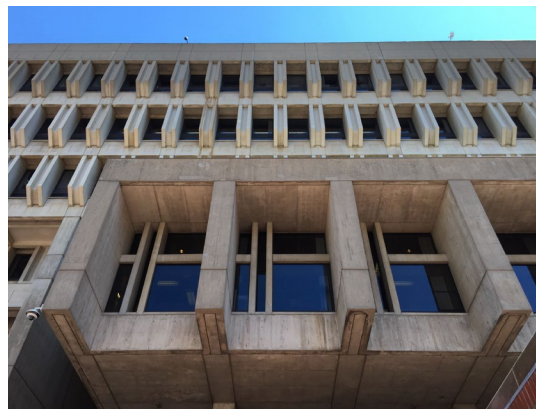
Hoods at the west-facing city council offices.
