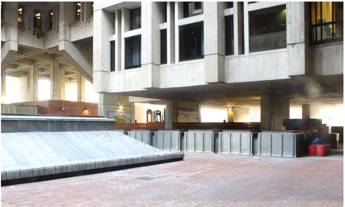
Views of the courtyard looking northeast showing the central skylight and bank of thirty-three skylights beyond.
