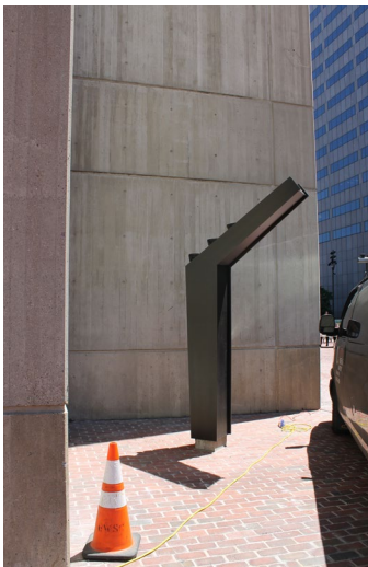
New sculptural style up-lighting at the building corners (May 23, 2018).
