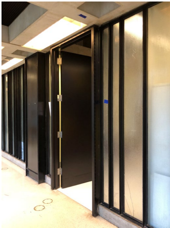
Cabinet inset into mullioned interior storefront.
