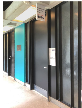
Entrance to the licensing hearing room showing newer hollow metal door and frame inserted into the mullioned interior storefront.
