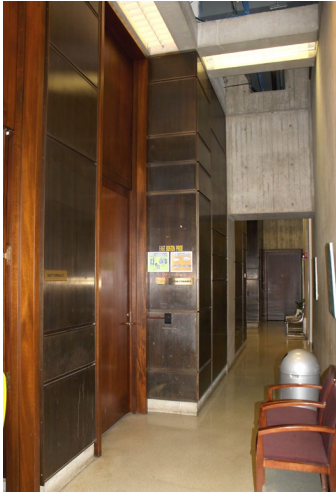
Typical bronze paneling conditions, city council corridor (June 21, 2018).
