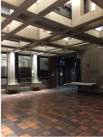
Vierendeel trusses and ceiling grid in the second-floor transaction area.
