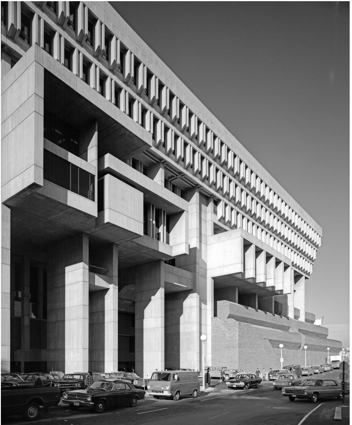
View of the east elevation from Congress Street.
