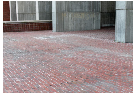
Top: Soldier course on the brick parapet walls nominally indicating the ground plane. (May 24, 2018).
