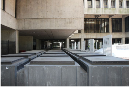
Bank of thirty-three skylights as seen in courtyard.
