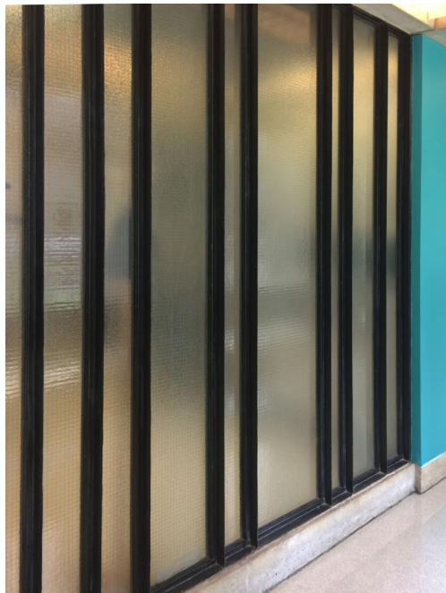
Example of corridor wall at the municipal level showing mullioned interior storefront with obscured wired plate glass.
