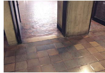
Brick to clay tile transition at the entry to the transaction area from the plaza lobby (March 29, 2018).
