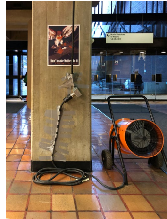
Supplementary heating with cords taped to the concrete.
