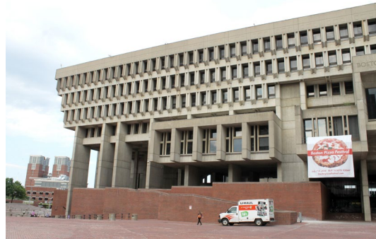
West (plaza side) elevation showing the brick mound (June 21, 2018).
