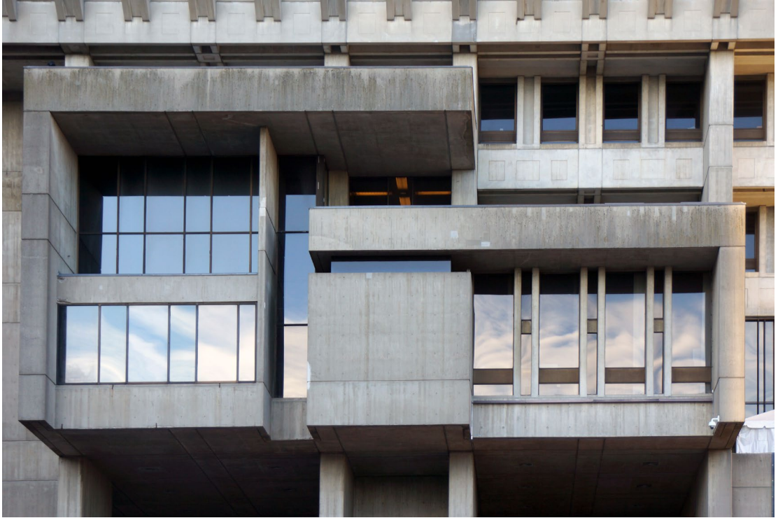
Glass in the ceremonial hood along the south facade (January 26, 2021).
