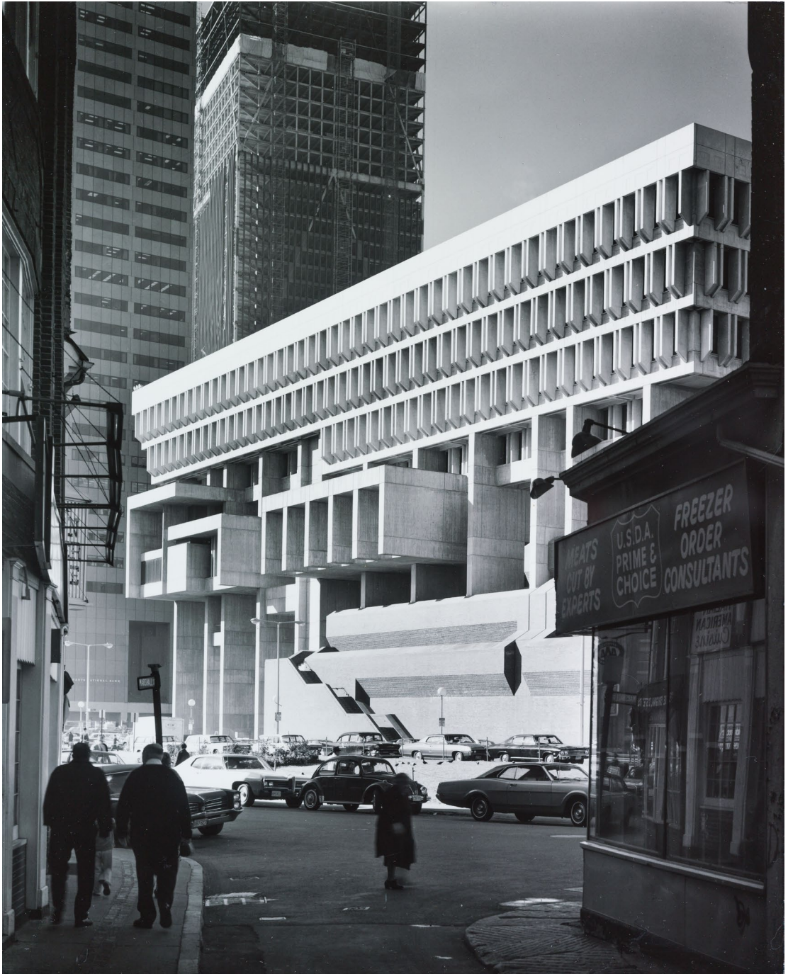
View of the east elevation from Union and Marshall Streets.
