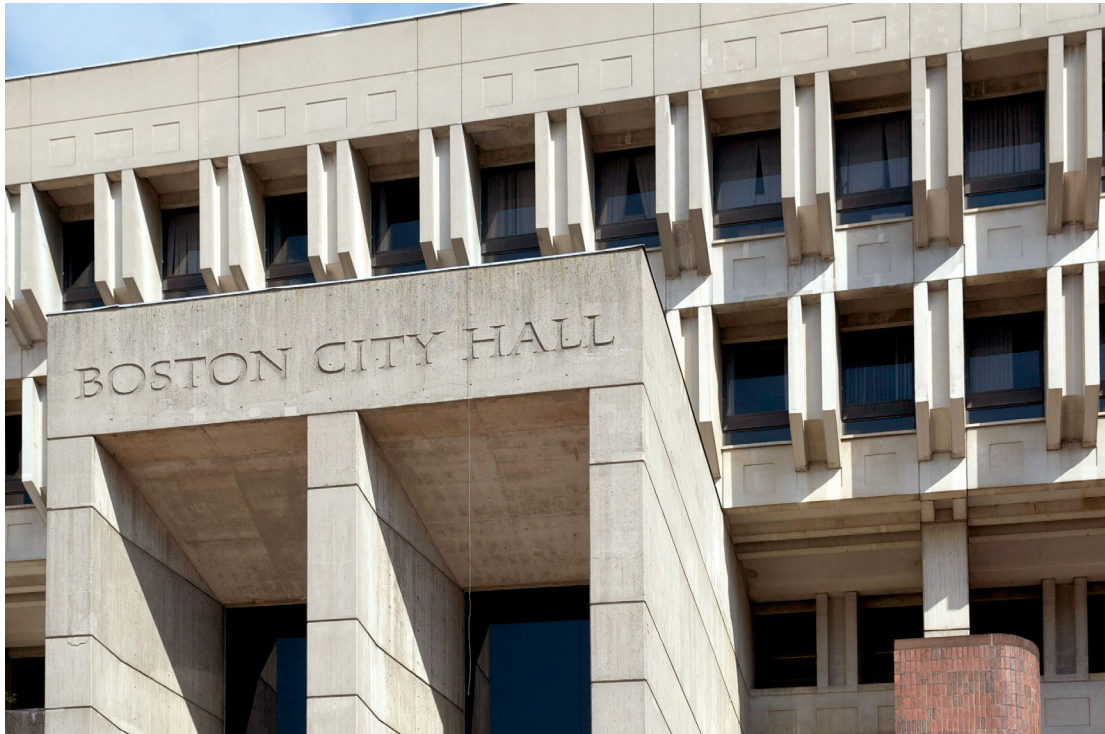
Cast-in-place concrete hood of the city council chamber with precast concrete fins and spandrels of the municipal levels beyond (September 5, 2009).
