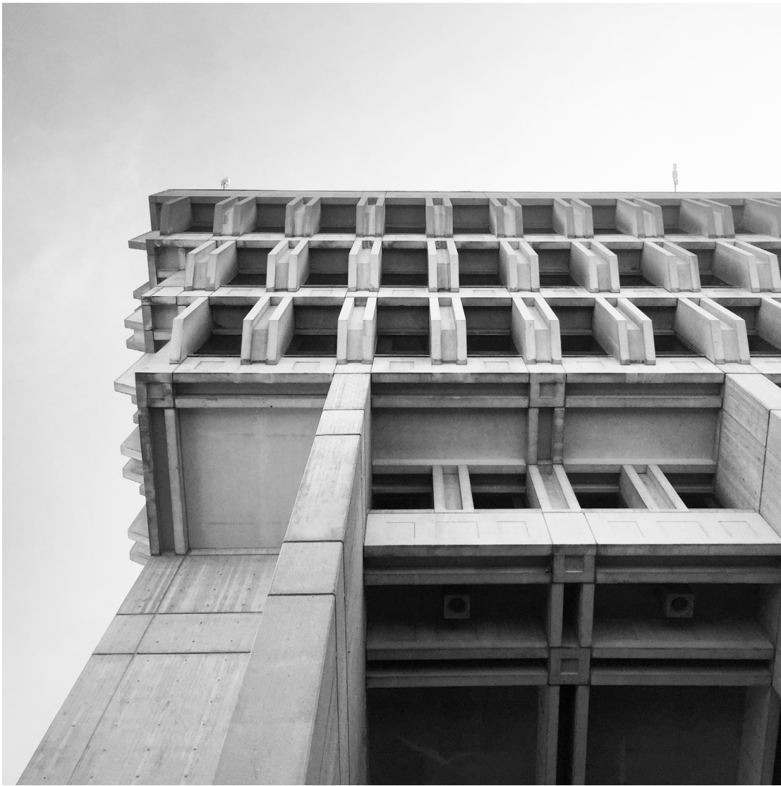
View of the southwest corner's municipal levels.
