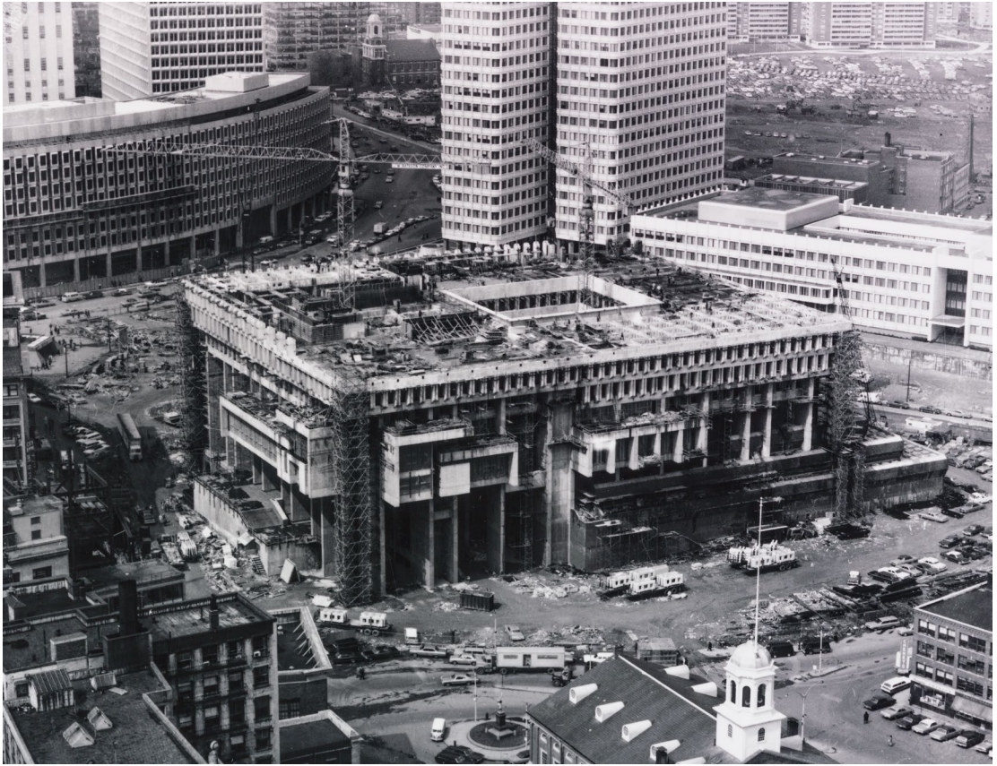
Top: Aerial view during construction.
