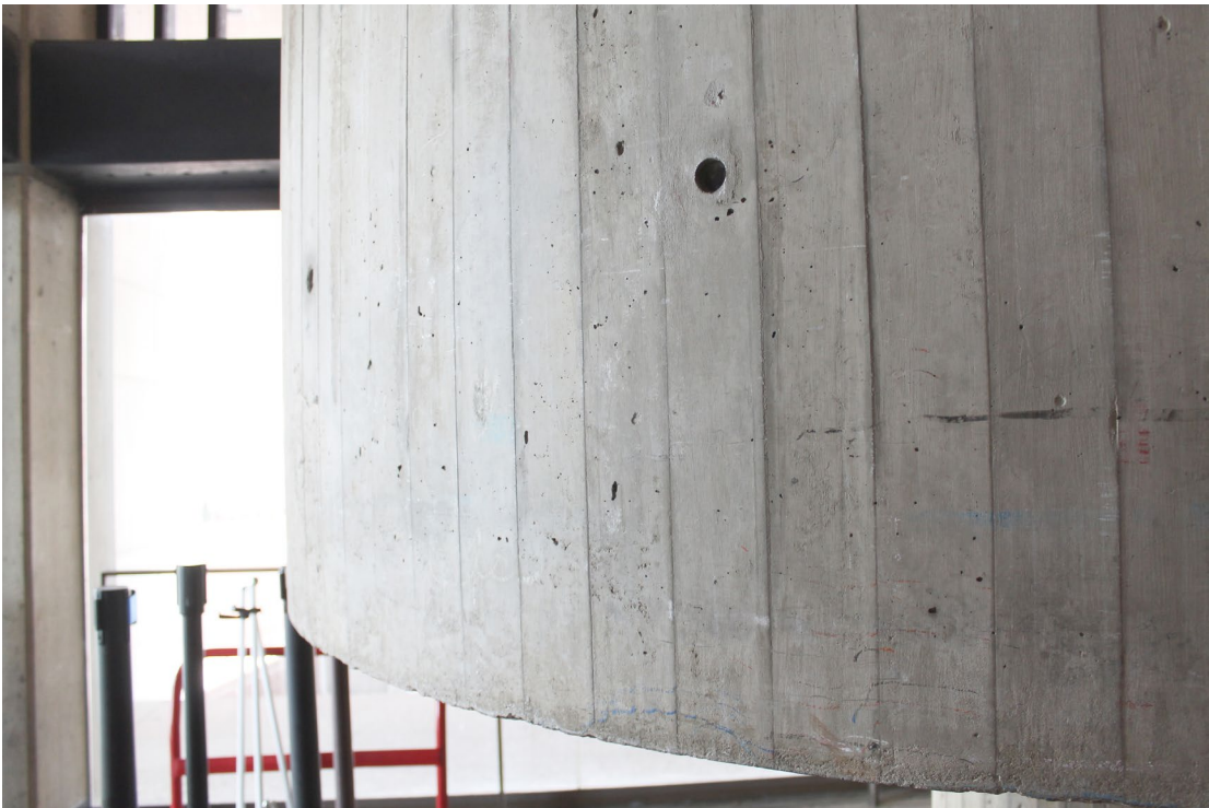
General conditions of interior concrete, shown at the mayor's stair (June 21, 2018).
