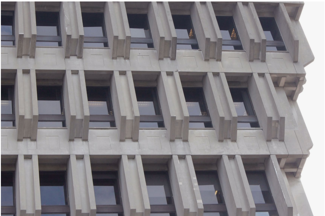
Typical window configuration at the municipal levels (June 21, 2018).
