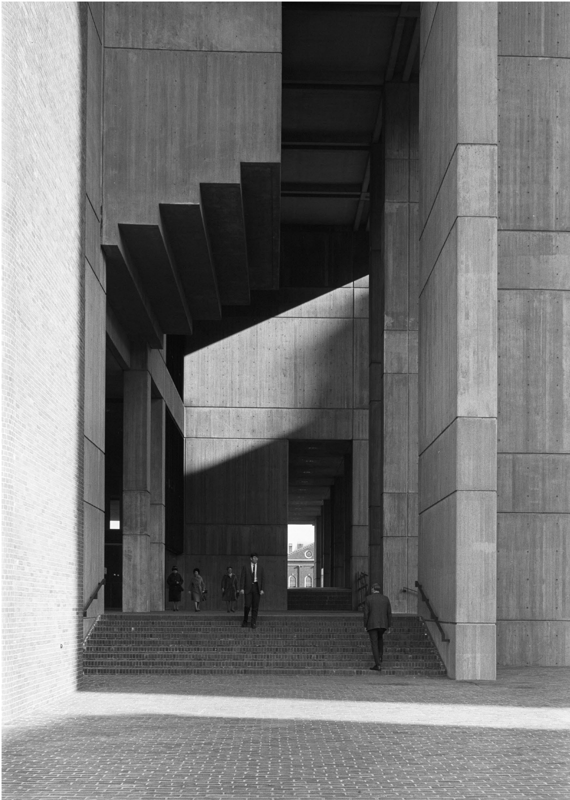
The entrance porch showing the underside of the stepped city council chamber.
