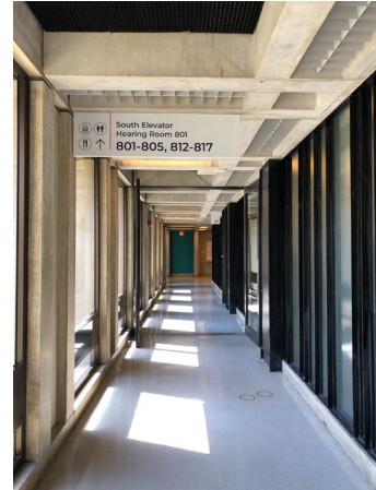
Typical municipal level corridor showing mullioned interior storefront and windows to the courtyard. New signage has been installed on the eighth floor.
