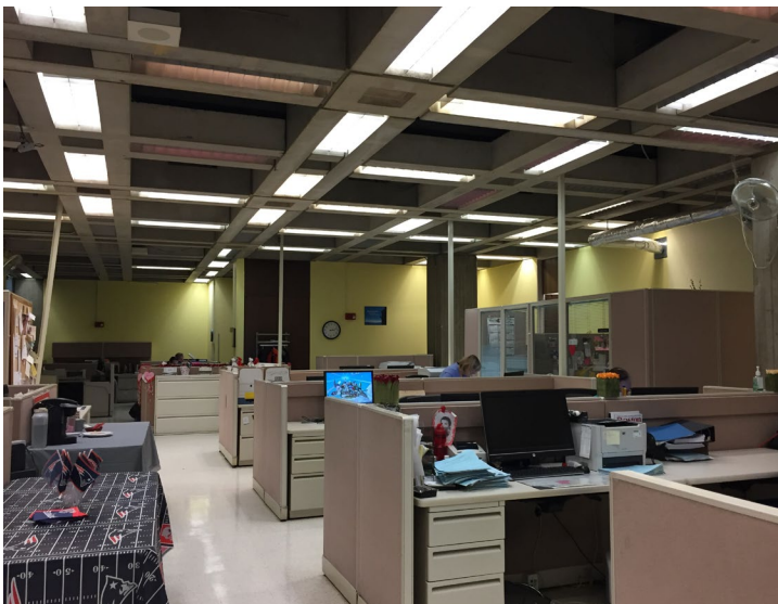
Second-floor office space showing power drops from the ceiling.
