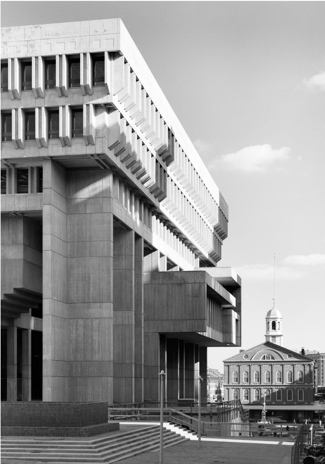
View of the southwest corner during construction of the plaza.
