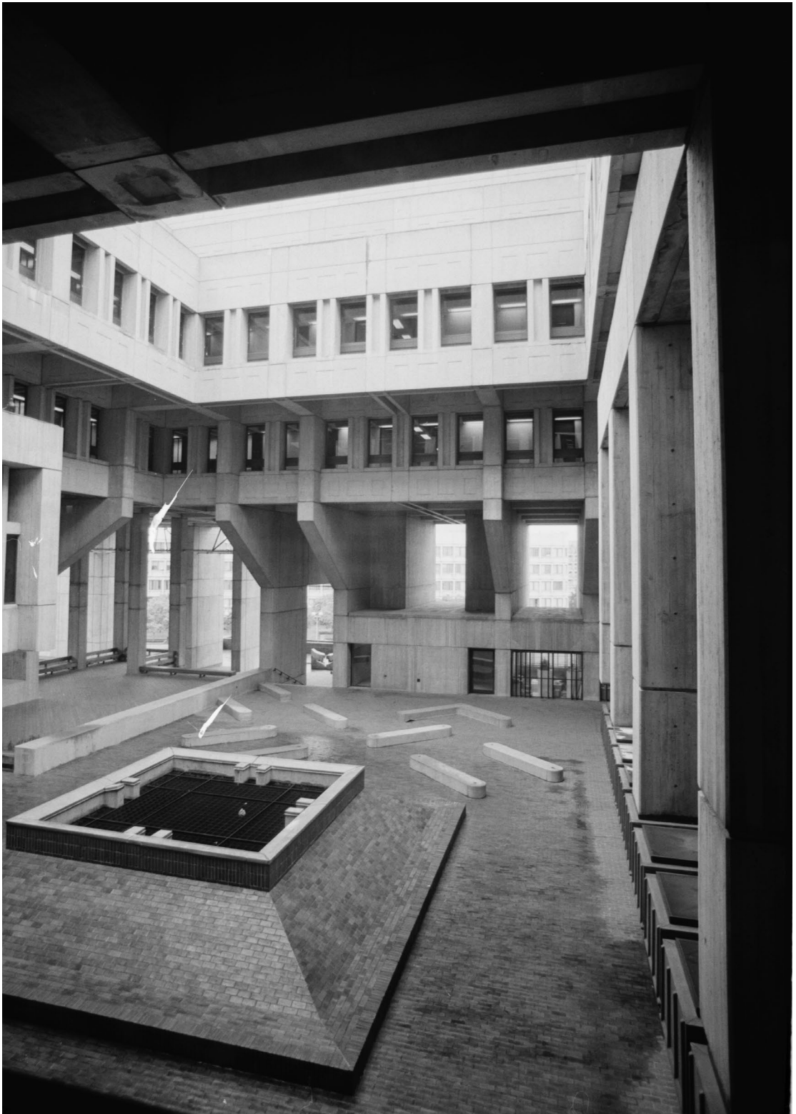
View of the courtyard and central skylight.
