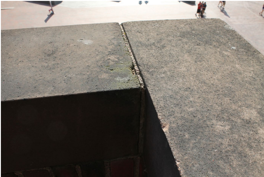
Brownstone with cementitious mortar joint (June 21, 2018).
