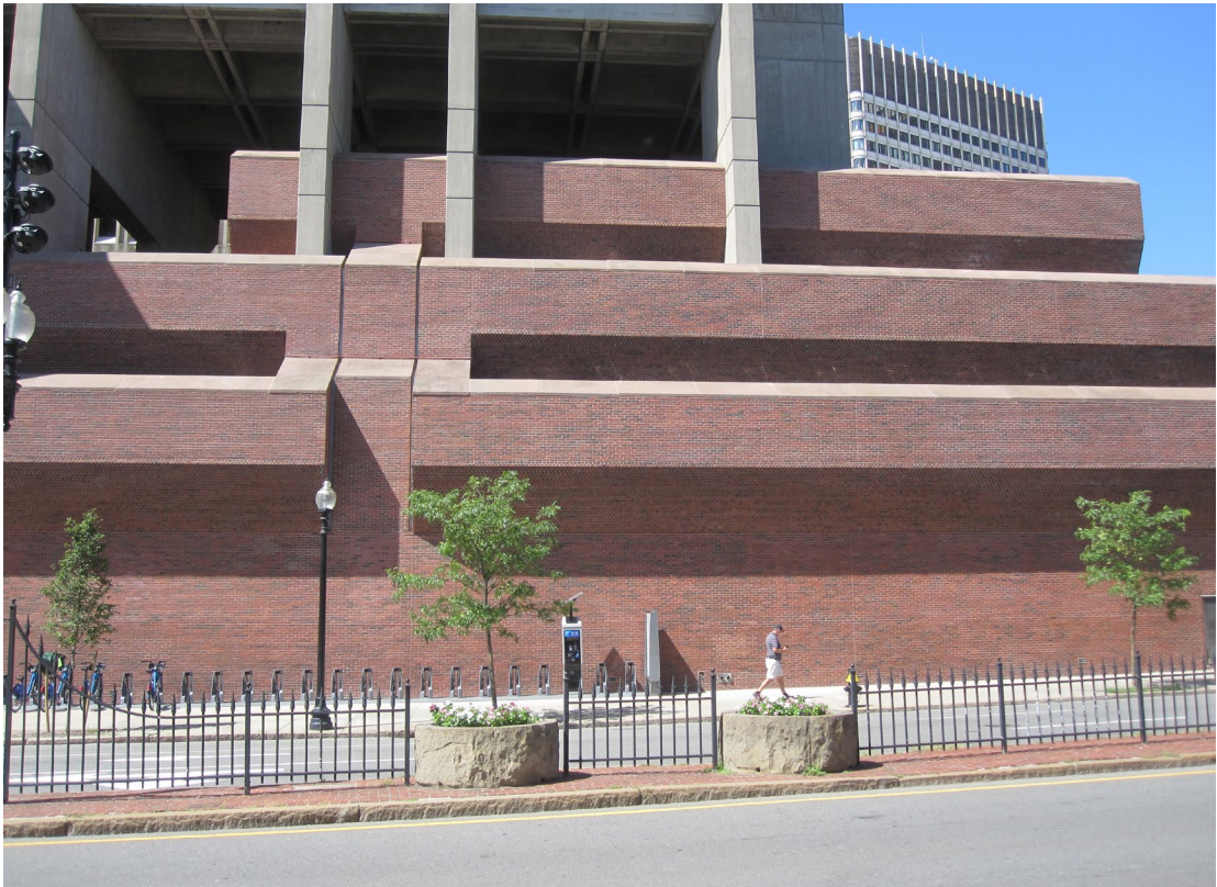
East (Congress Street) elevation showing the terraced brick mound (August 26, 2019).
