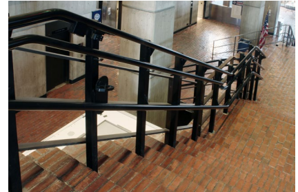
Rail-mounted lift on the monumental stair.
