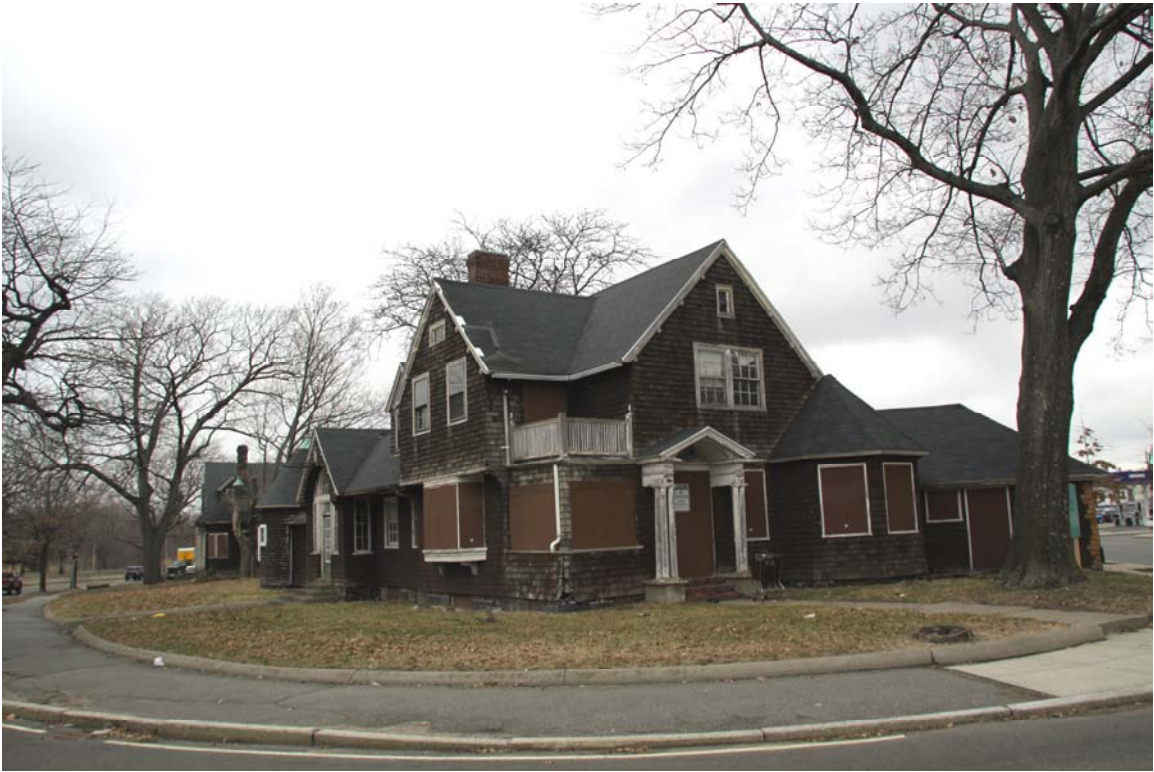
Figure 13. Southwestern and northwestern elevations of Superintendent's Residence (D).
