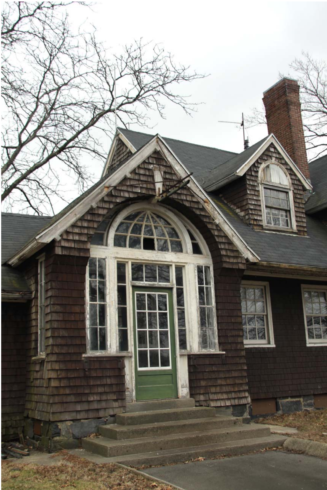
Figure 18. Metropolitan Park Commission Police Headquarters (E), detail of entrance.
