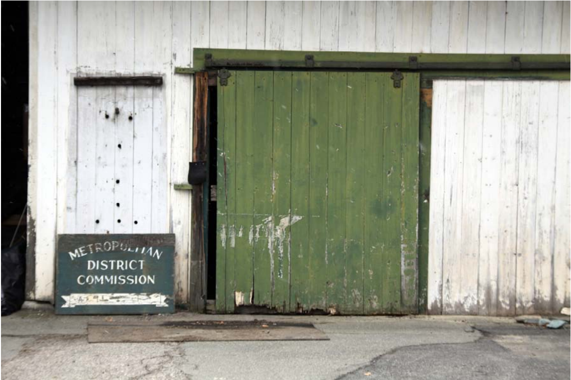
Figure 9. Detail of sliding barn-style door, courtyard-facing elevation of South Shed (C).
