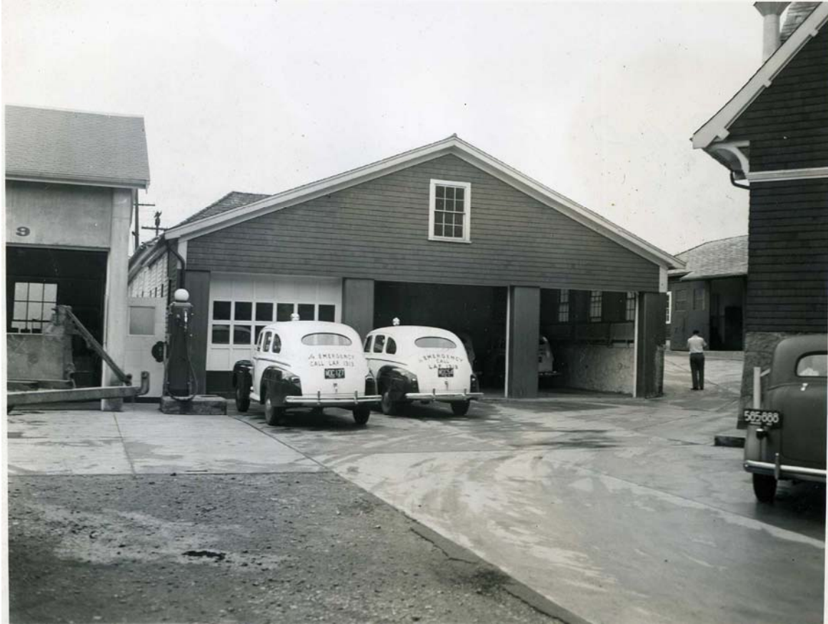
Figure 33. Northern elevation of Garage, 1941 (Courtesy DCR Archives, Metropolitan District Commission Parks Buildings Photographic Survey Collection, 1941).
