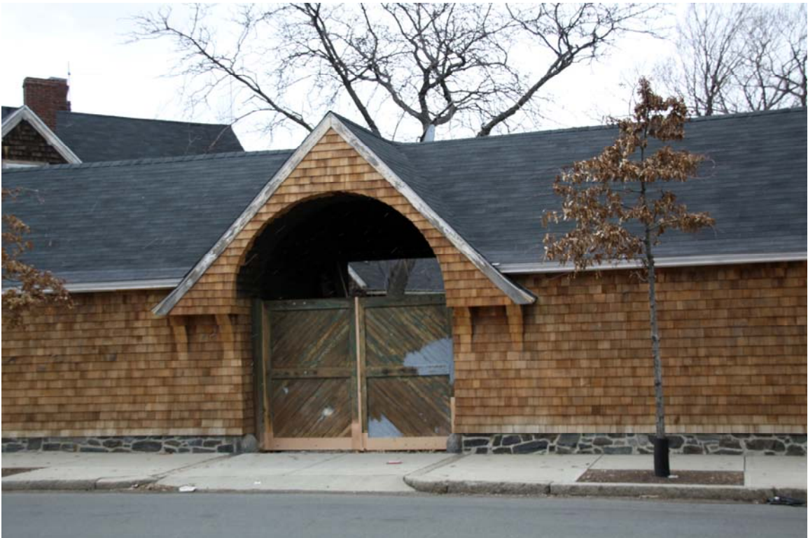
Figure 12. South Shed (C), view from Western Avenue. Detail of entrance portal.
