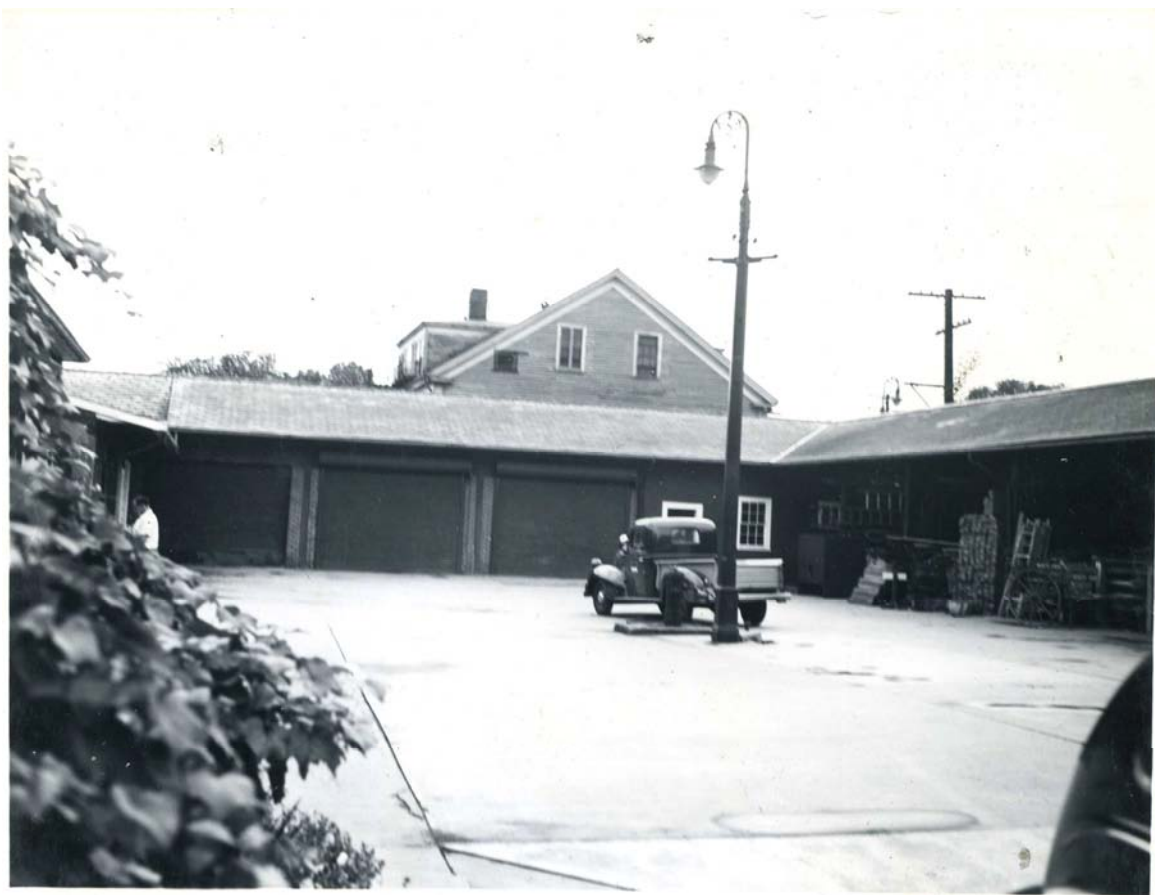
Figure 34. View of courtyard-facing elevations of East Shed and South Shed, 1941 (Courtesy DCR Archives, Metropolitan District Commission Parks Buildings Photographic Survey Collection, 1941).
