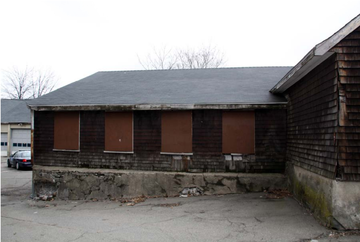
Figure 5. Western elevation of Garage (A).
