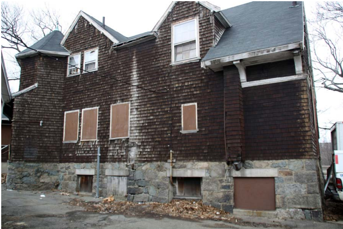
Figure 22. Metropolitan District Commission Stable and Police Station (F), southeastern elevation.
