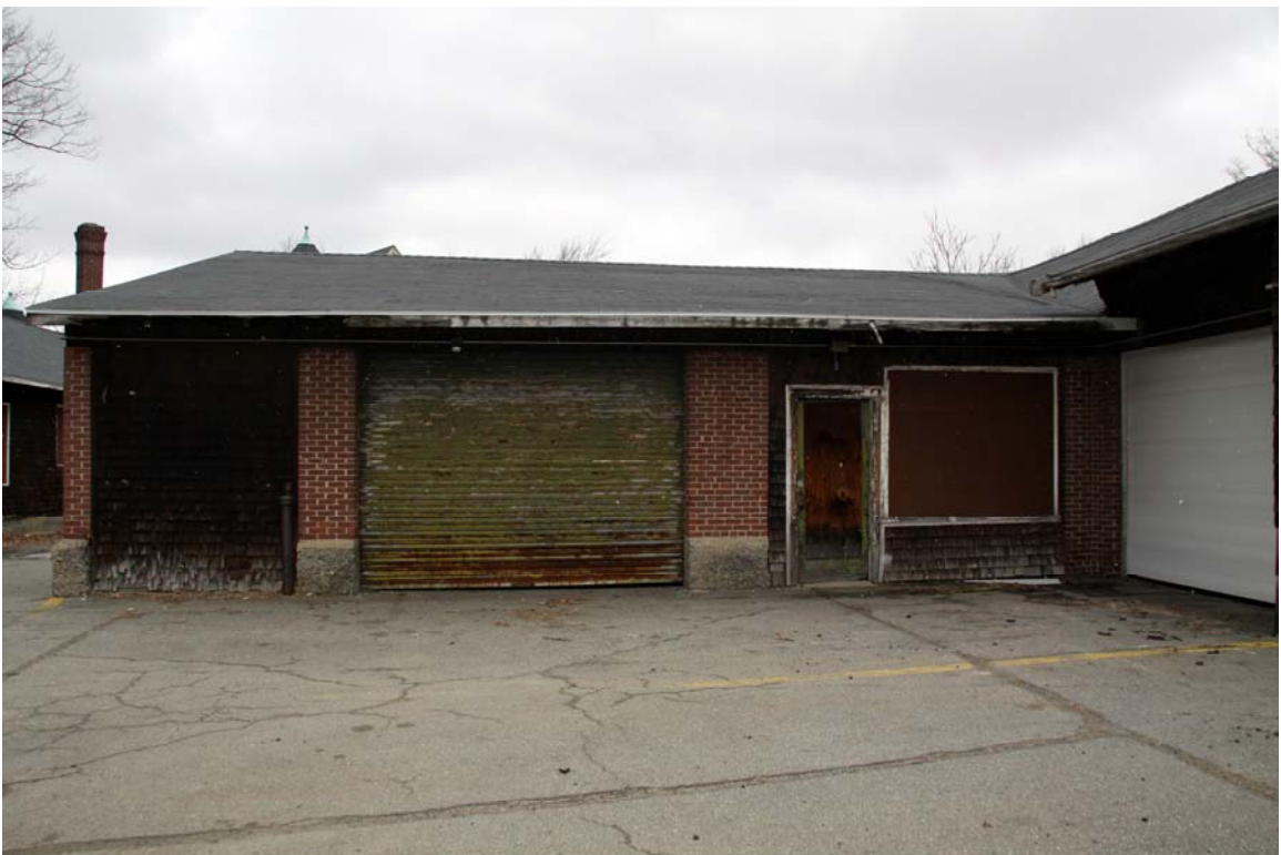
Figure 6. Southern elevation of East Shed (B).
