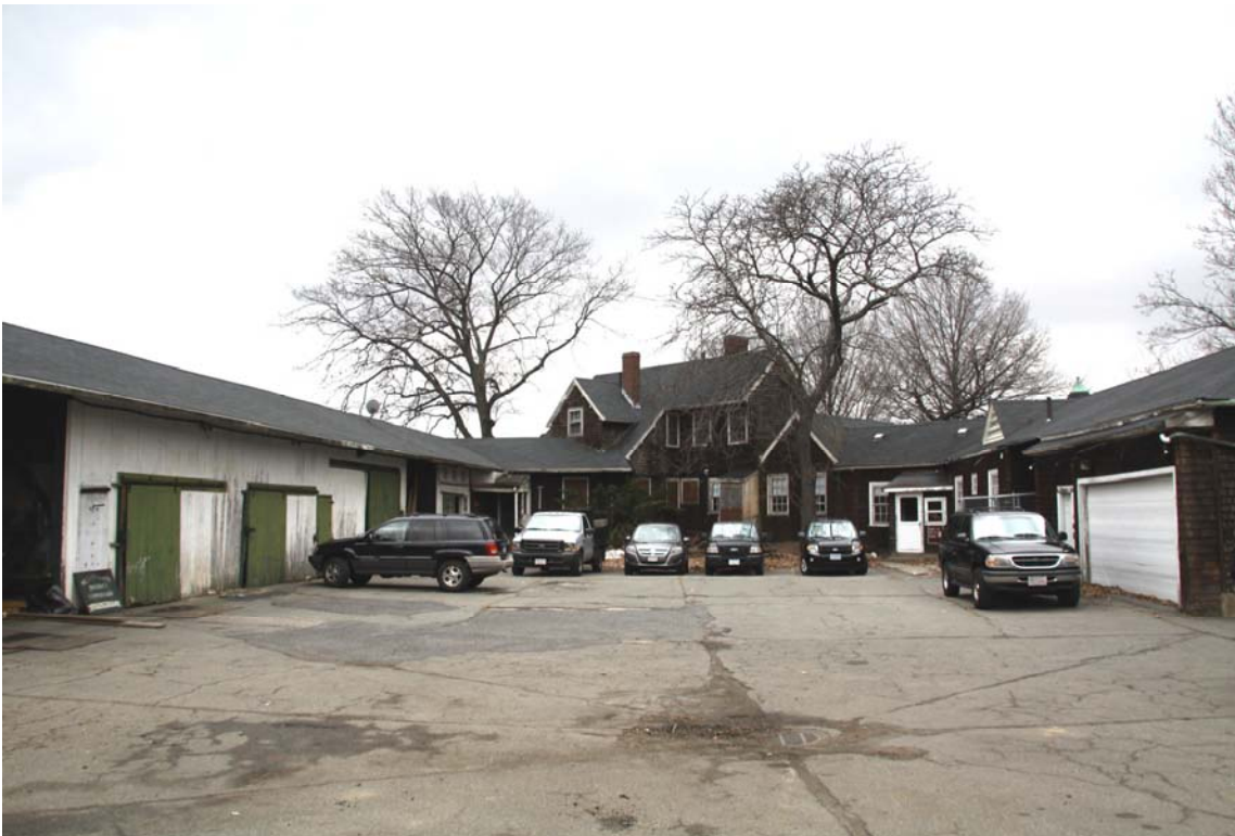
Figure 24. View of courtyard, facing west.
