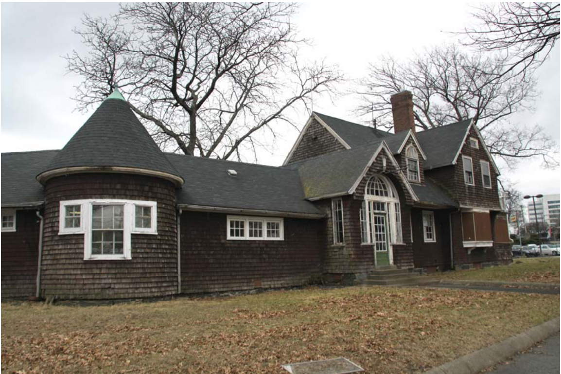
Figure 17. Northwestern elevation of Metropolitan Park Commission Police Headquarters (E), with Superintendent's Residence (D) beyond.
