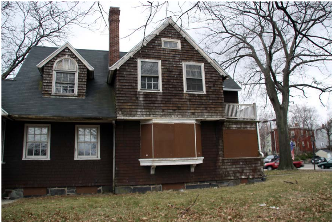
Figure 14. Northwestern elevation of Superintendent's Residence (D).
