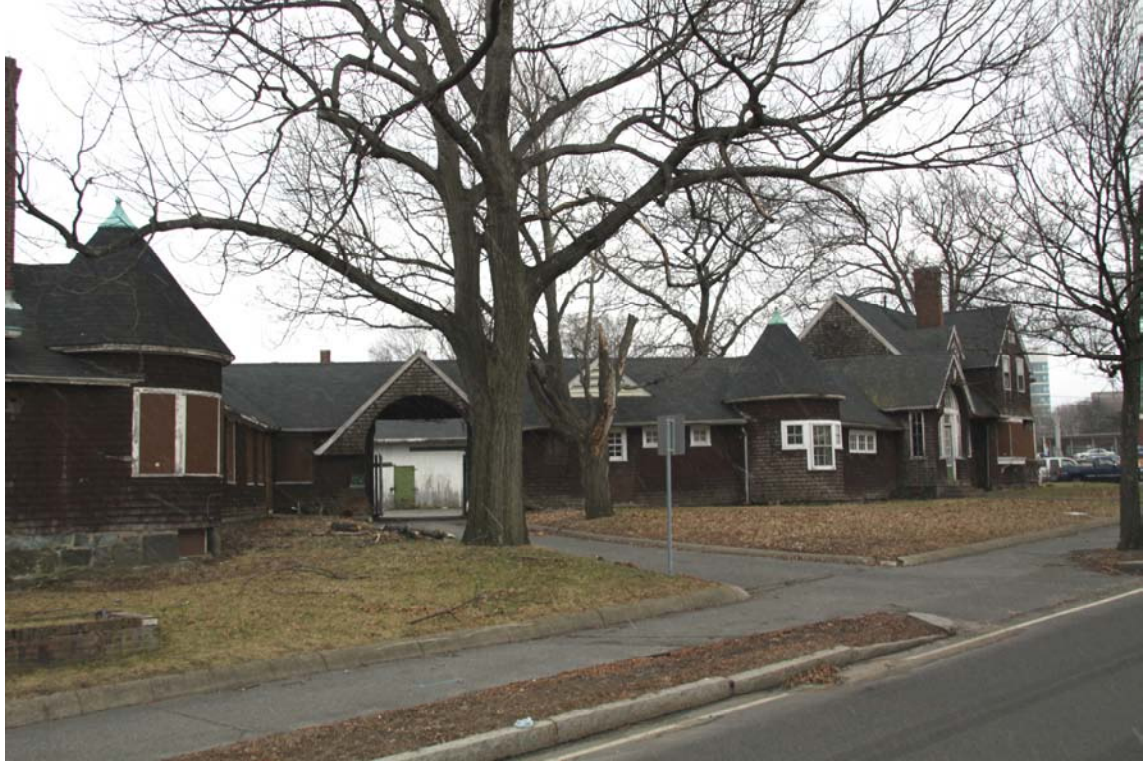
Figure 19. Northern elevation, Metropolitan Park Commission Police Headquarters (E).
