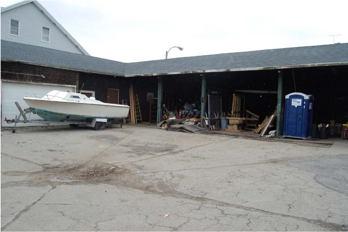
Figure 7. Courtyard-facing elevations of East Shed (B) and South Shed (C).
