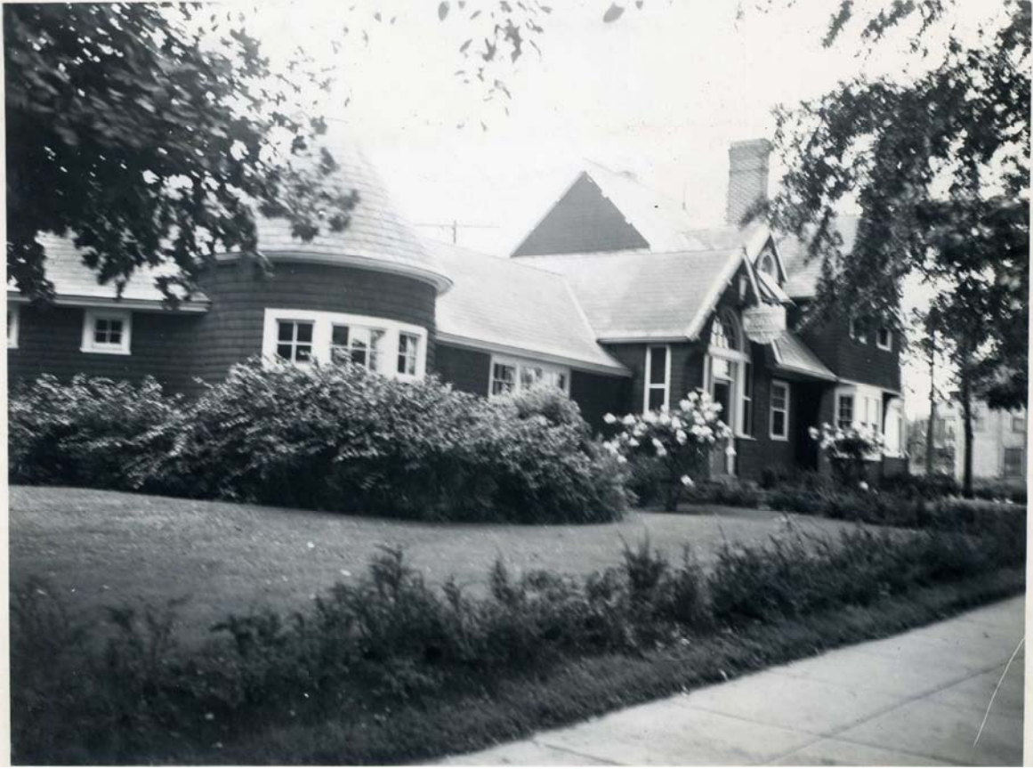
Figure 36. Metropolitan Park Commission Police Headquarters and Superintendent's Residence, 1941 (Courtesy DCR Archives, Metropolitan District Commission Parks Buildings Photographic Survey Collection, 1941).
